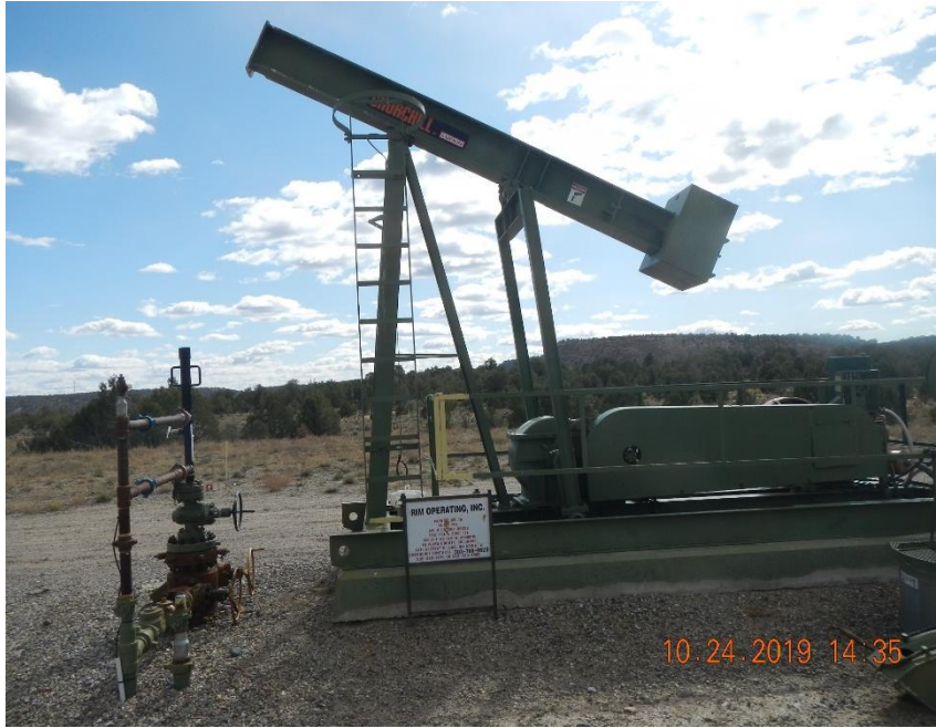
Dismantled pump jack at the Payne C #1A. Plunger lift in use on well.
