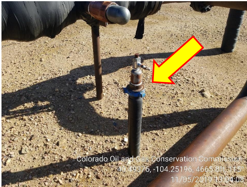
Photo 5 – Unmarked 3" Risers
