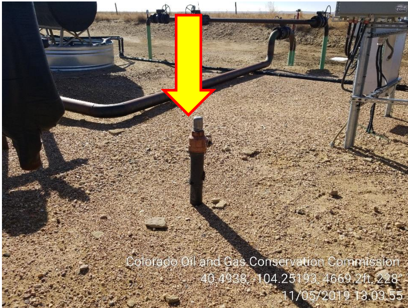
Photo 3 – Unmarked 2" Risers
