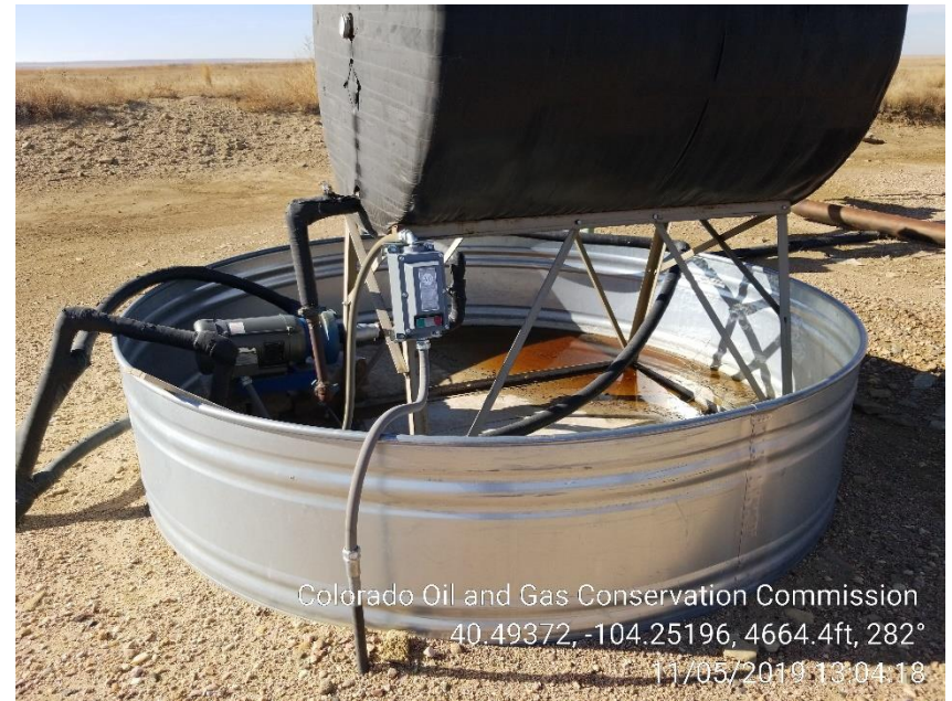
Photo 8 – Containment is vulnerable to wildlife intrusion.
