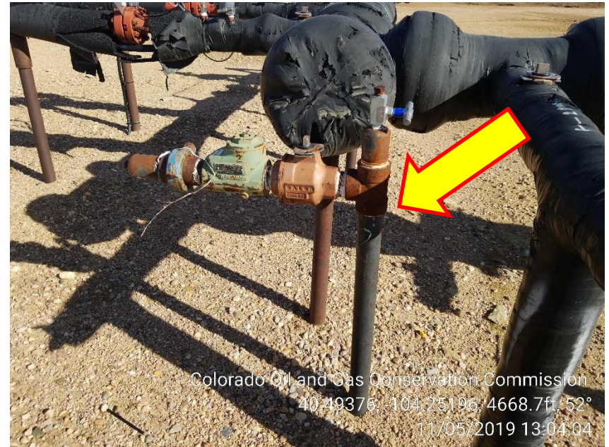
Photo 4 –Unmarked 2" Risers
