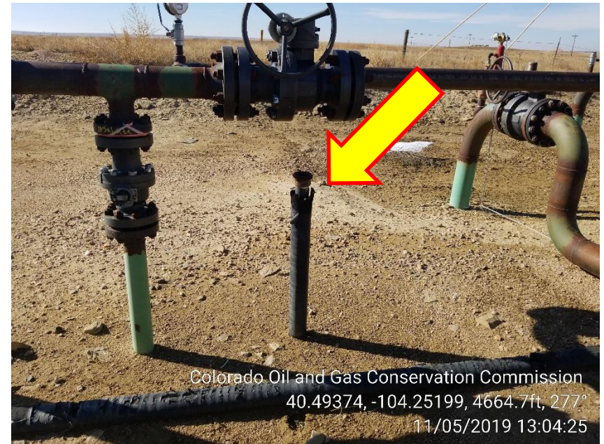
Photo 6 – Unmarked 2" Risers
