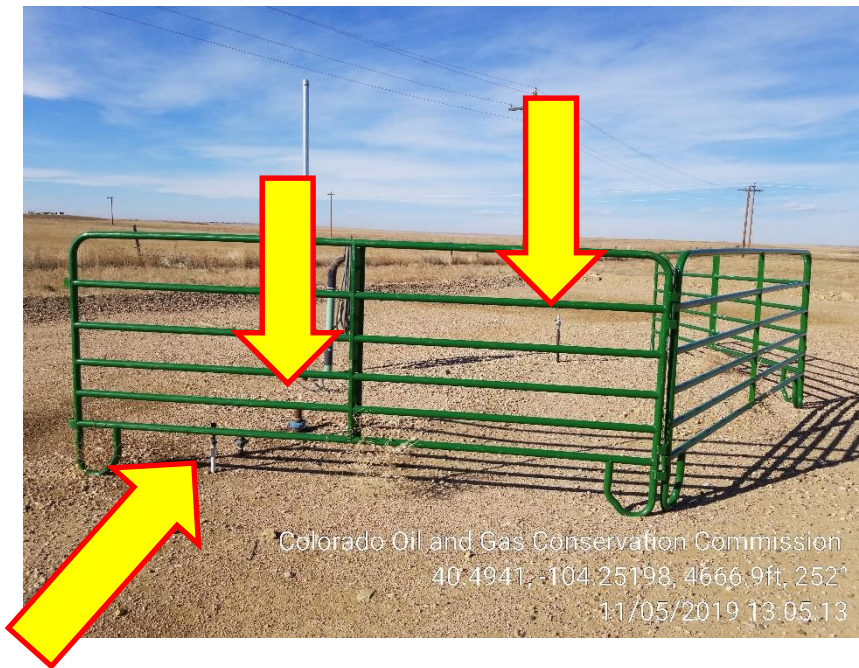
Photo 7 – Unmarked 1" and 2" Risers
