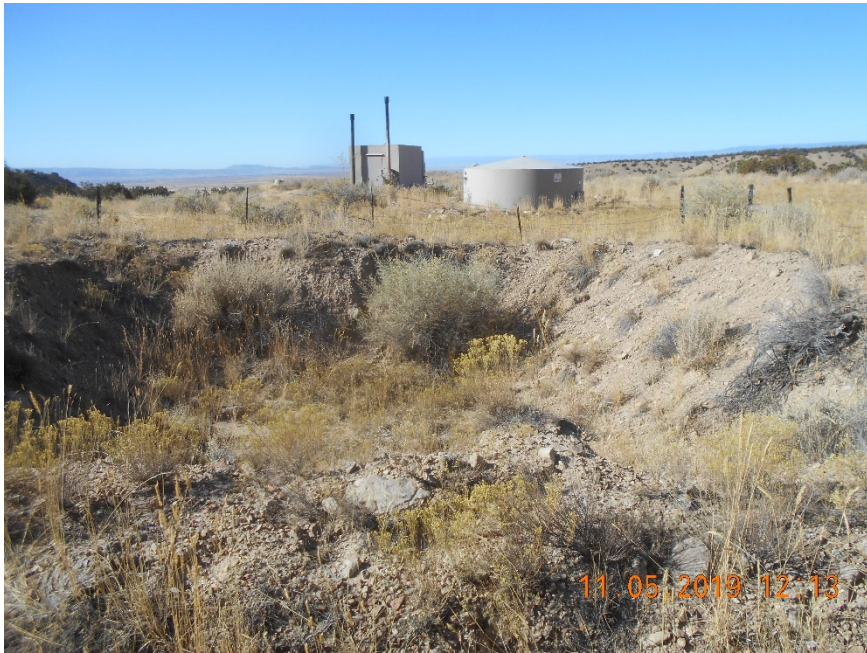
Blowdown pit with fence
