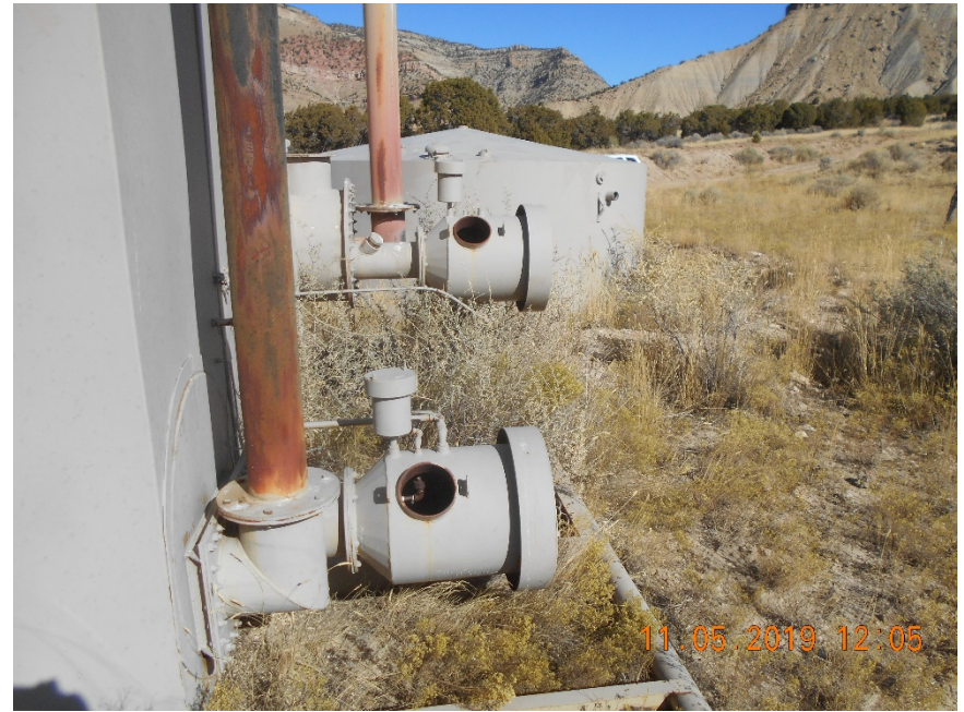
Separator burners with open access.
