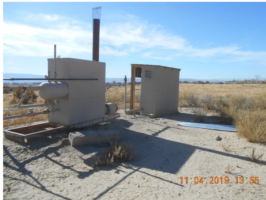
Trash and Meter housing panels/doors blown off.
