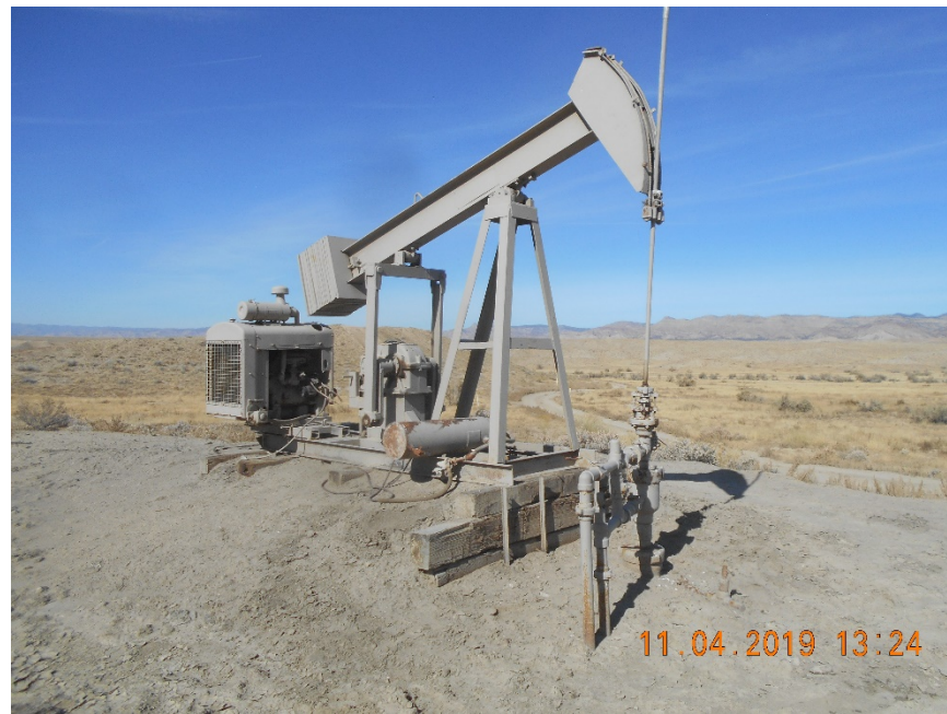
Wellhead with Pump jack.
