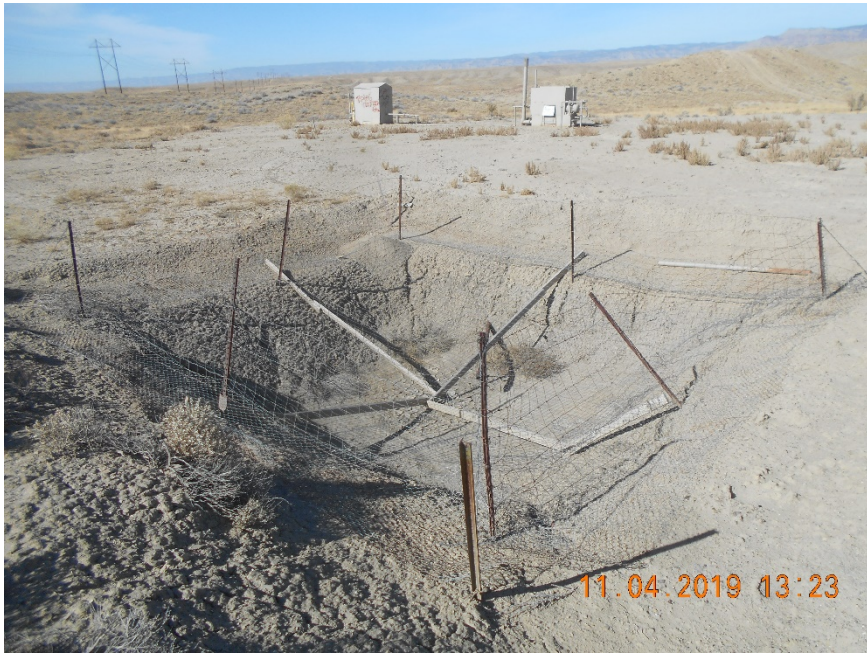
Blowdown pit with fence and netting.
