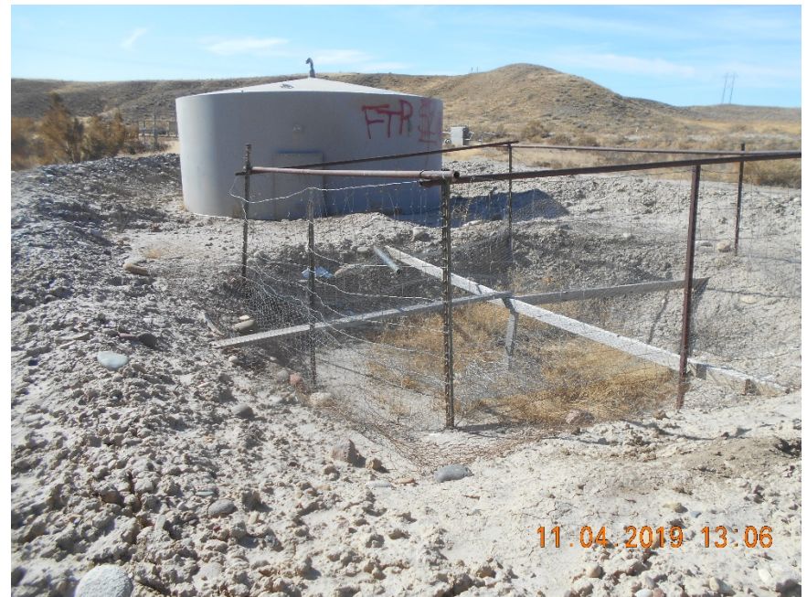
Produced water tank and blowdown pit with fence and netting.
