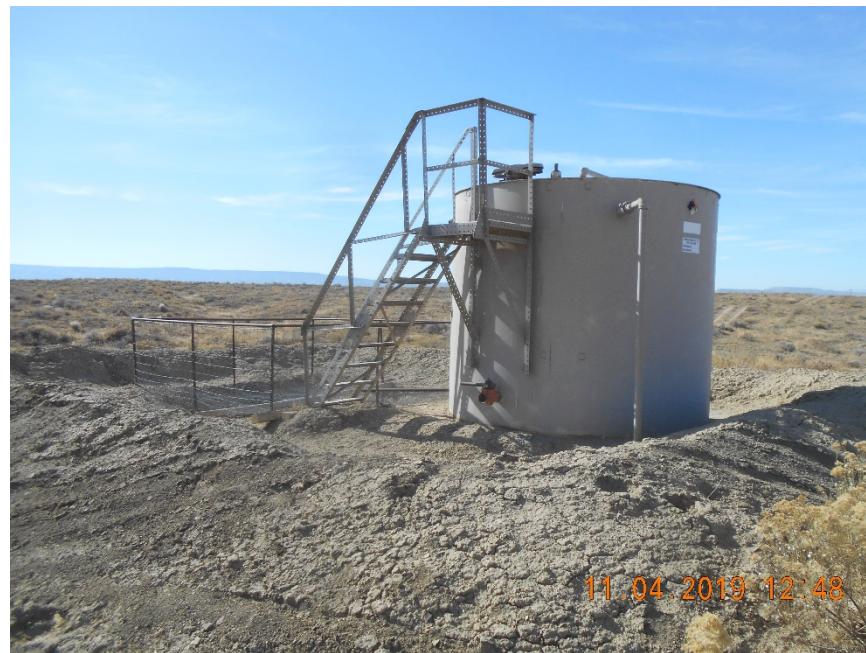
Produced water tank with faded and peeling labels.
