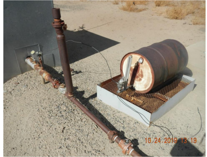
Secondary containment for chemical container.
