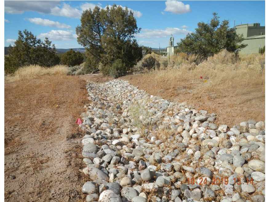
Rip rap run down along northern edge of location.
