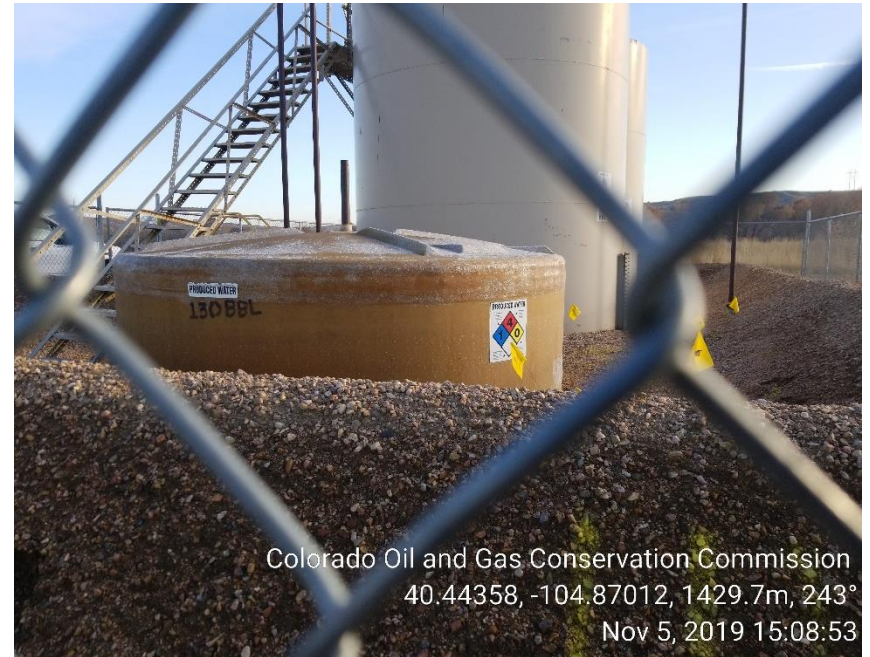
Photo 4: Tank NOT anchored
