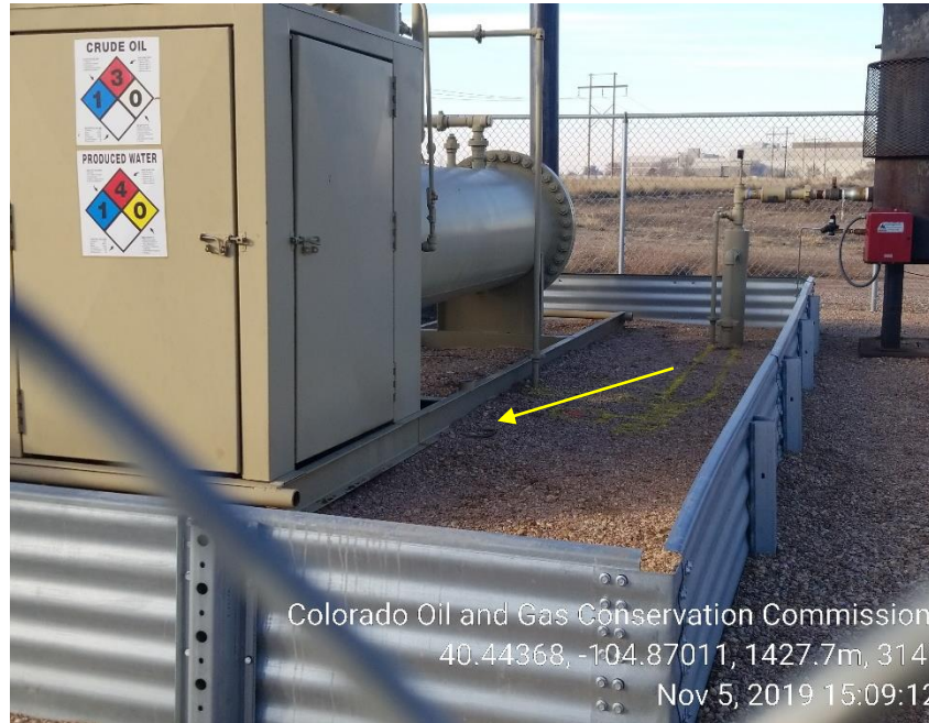
Photo 5: Separator NOT anchored
