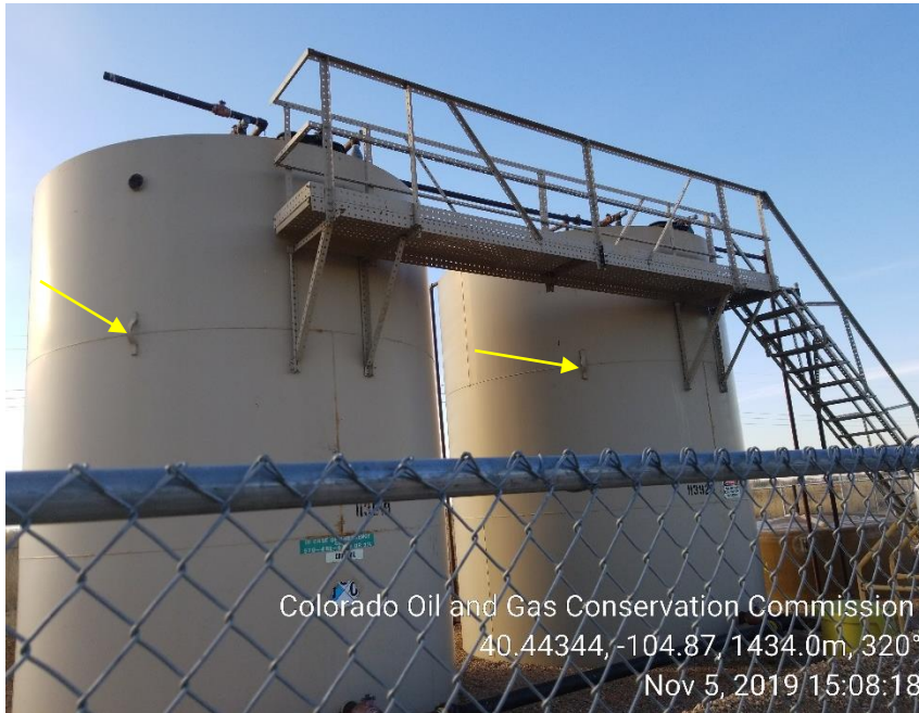
Photo 3: Tanks NOT anchored
