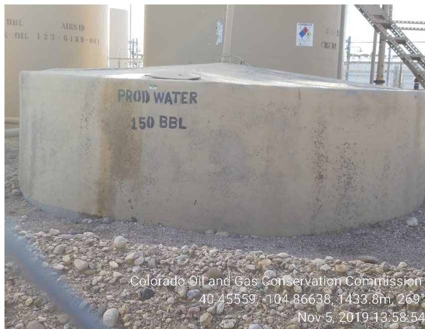
Photo 5: No NFPA placard/tank NOT anchored
