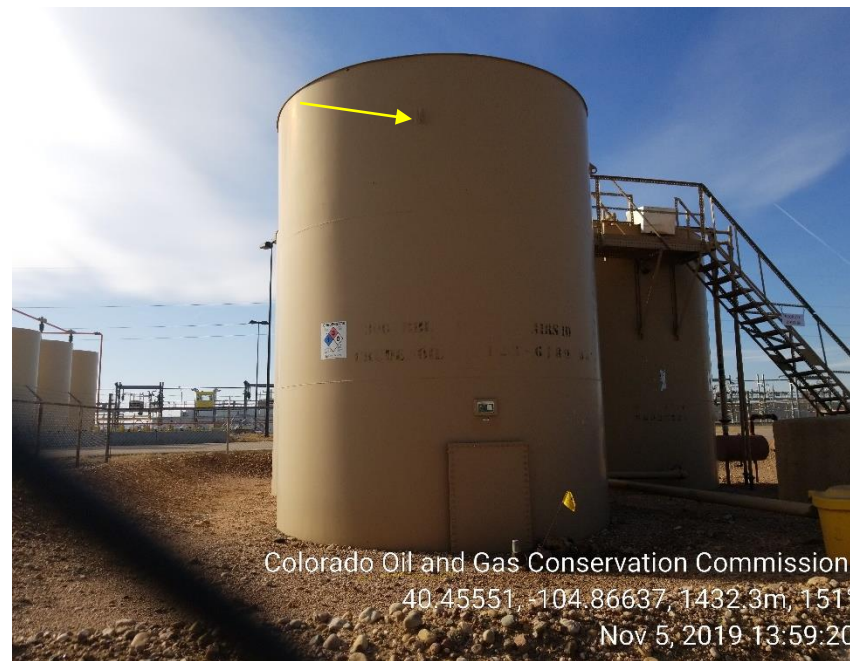
Photo 6: Tank NOT anchored
