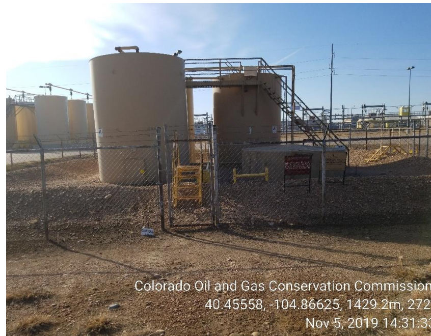
Photo 4: Tank Battery/inadequate berms
