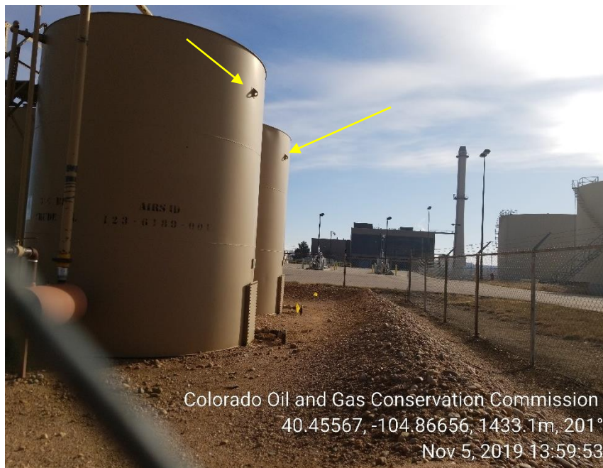
Photo 7: Tanks NOT anchored
