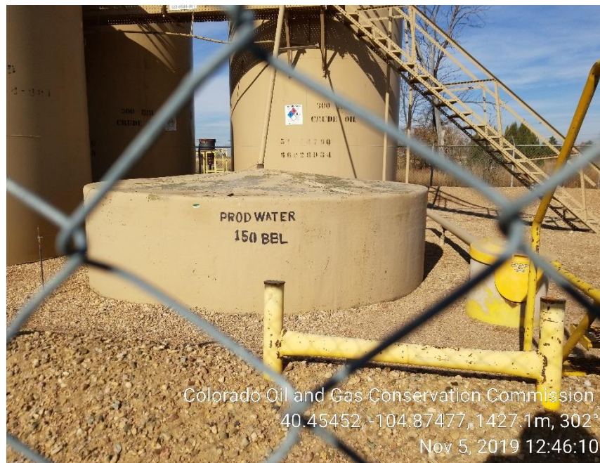
Photo 11: No NFPA placard on h2o tank
