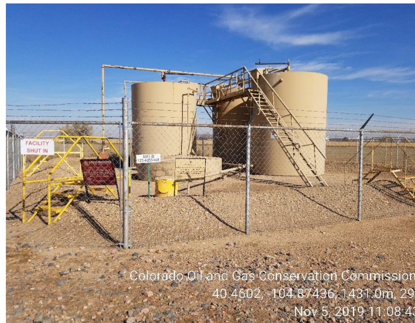
Photo 6: Tank Battery/ inadequate berm (earth)
