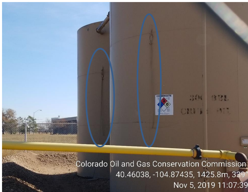
Photo 9: Tanks anchored
