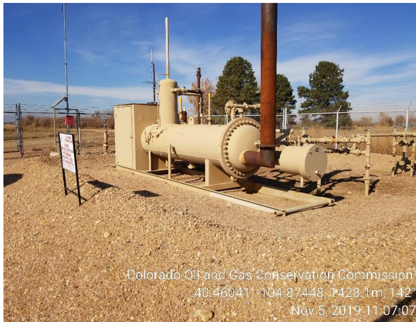
Photo 7: Separator NOT anchored
