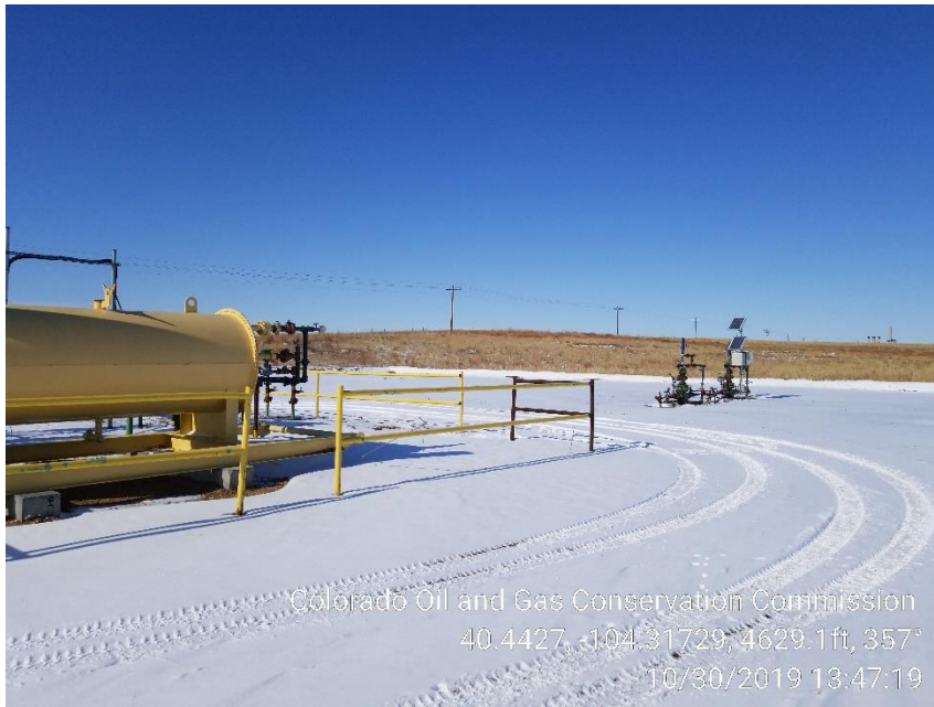
Photo 1 – 3349BH2, 4841BH2 - Wellheads
