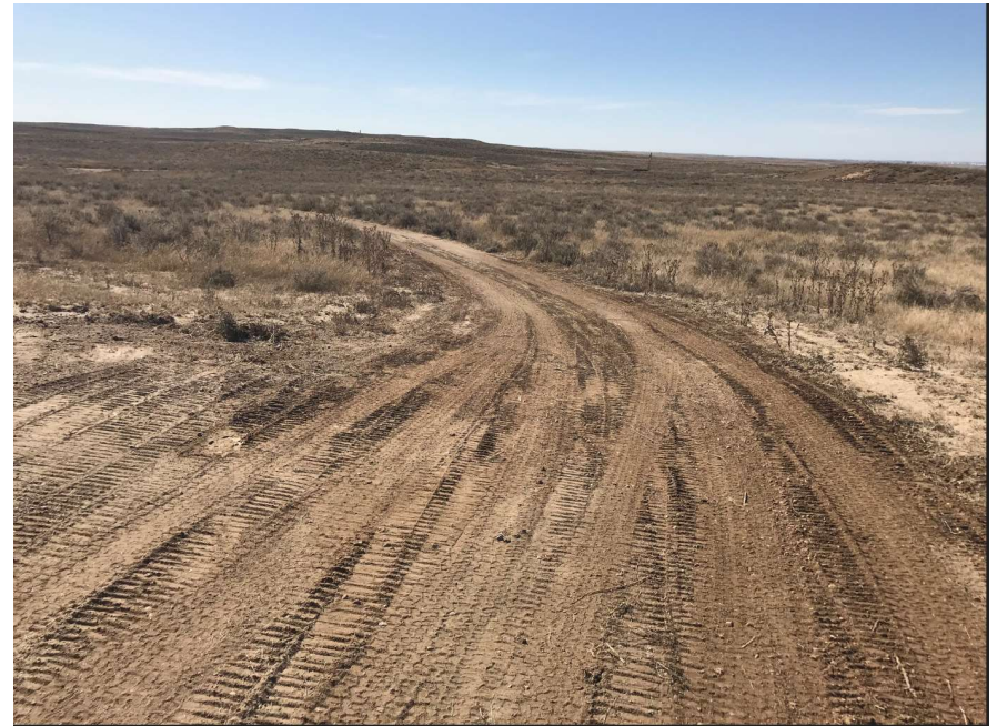
Photo NBL5. Erosion back-filled and compacted roadbed.
