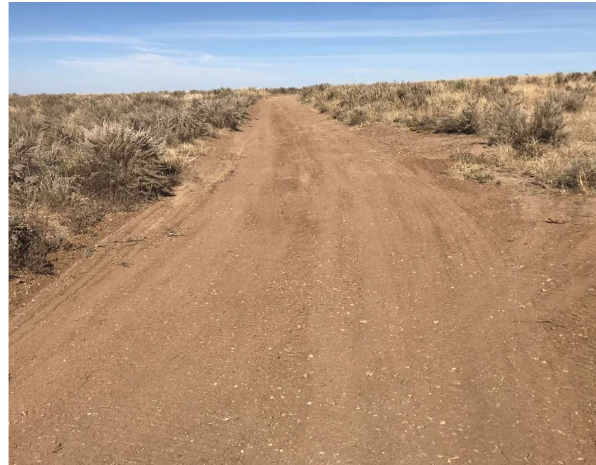
Photo NBL1. Erosion back-filled and compacted roadbed.
