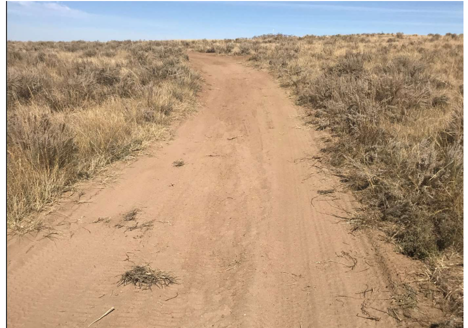
Photo NBL2. Erosion back-filled and compacted roadbed.
