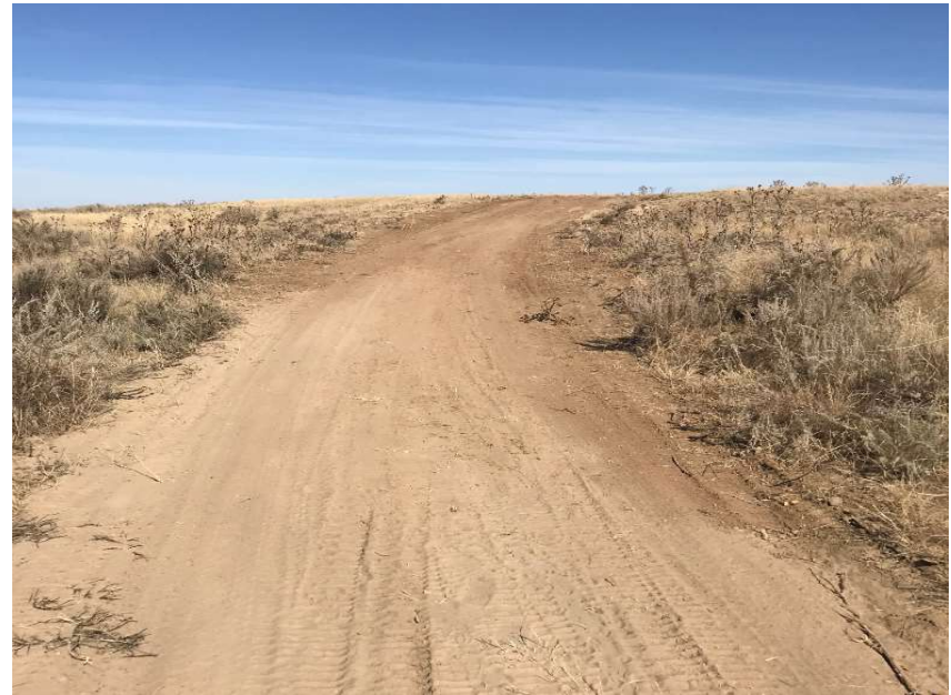
Photo NBL4. Filtrex installed outside fence. Erosion repaired, and sloped compacted and tracked.
