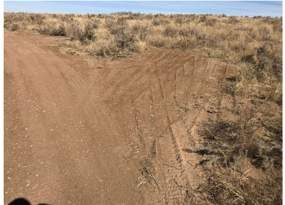
Photo NBL3. Erosion back-filled and compacted roadbed.
