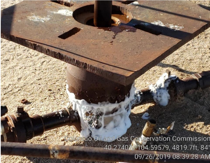
Photo #2 Active leak at the casing collar. On 9/26/19
