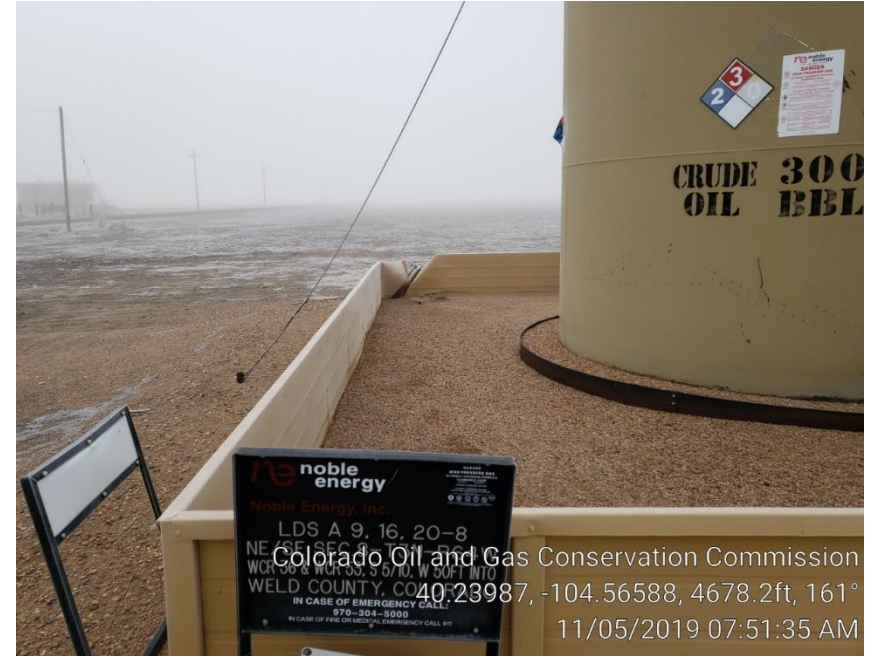
Photo #2 picture taken on the north side, Berm wall is Mangled up. 11/5/19
