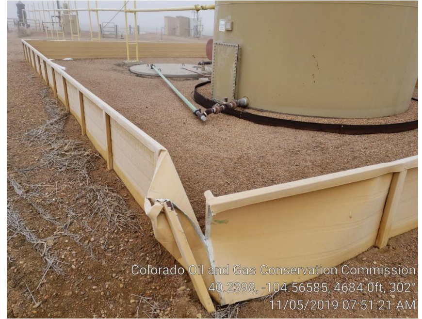
Photo #4 Picture taken from the SE corner, Berm wall is Mangled up. On 11/5/19
