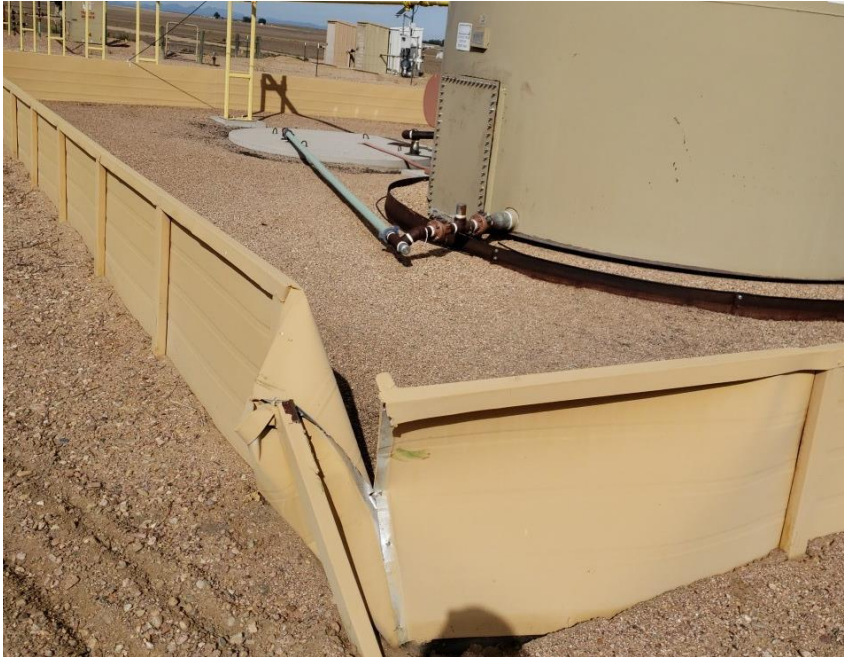
Photo #3 Picture taken from the SE corner, Berm wall is Mangled up. On 9/23/19
