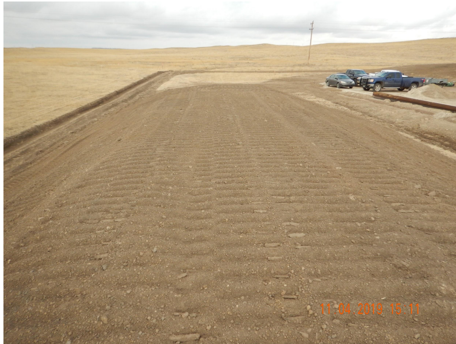
Photo 4. Photo taken from the western location, facing North. Photo illustrates the topsoil stockpile which has been temporarily stabilized with equipment tracking.
