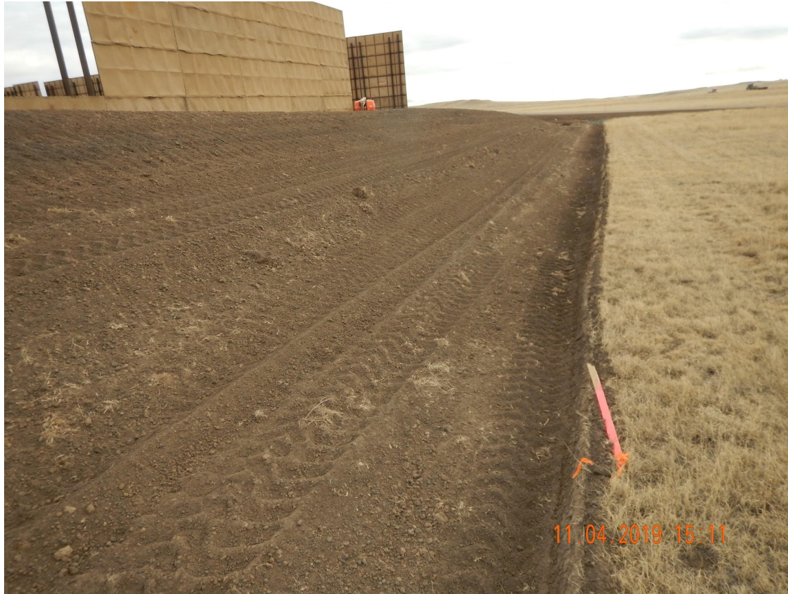
Photo 6. Photo taken from the western perimeter of location, facing South. Photo illustrates a shallow ditch BMP along the western location. This ditch BMP would not be considered installed to a sufficient depth.
