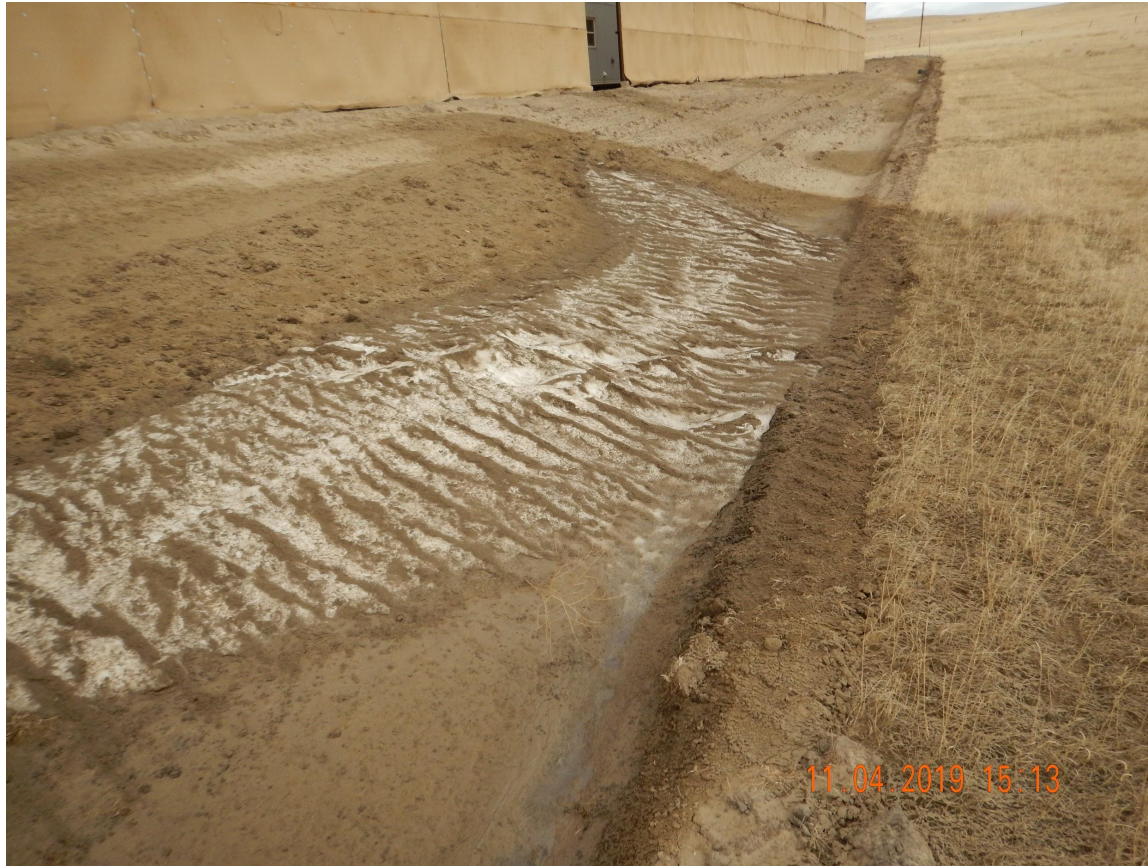
Photo 9. Photo taken from the southern perimeter of location, facing East. Photo illustrates sediment accumulation within the shallow ditch BMP. Also, Operator shall stabilized the unconsolidated fill material along the southern location as this is susceptible to wind and water erosion.
