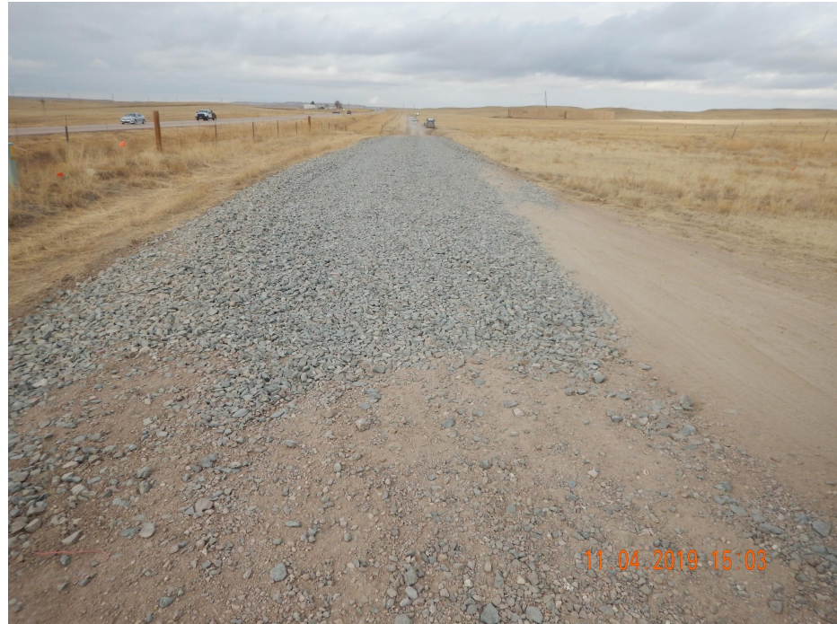
Photo 2. Photo taken from the entrance of location off HWY 85, facing North. Photo illustrates Operator has installed a vehicle tracking device BMP.
