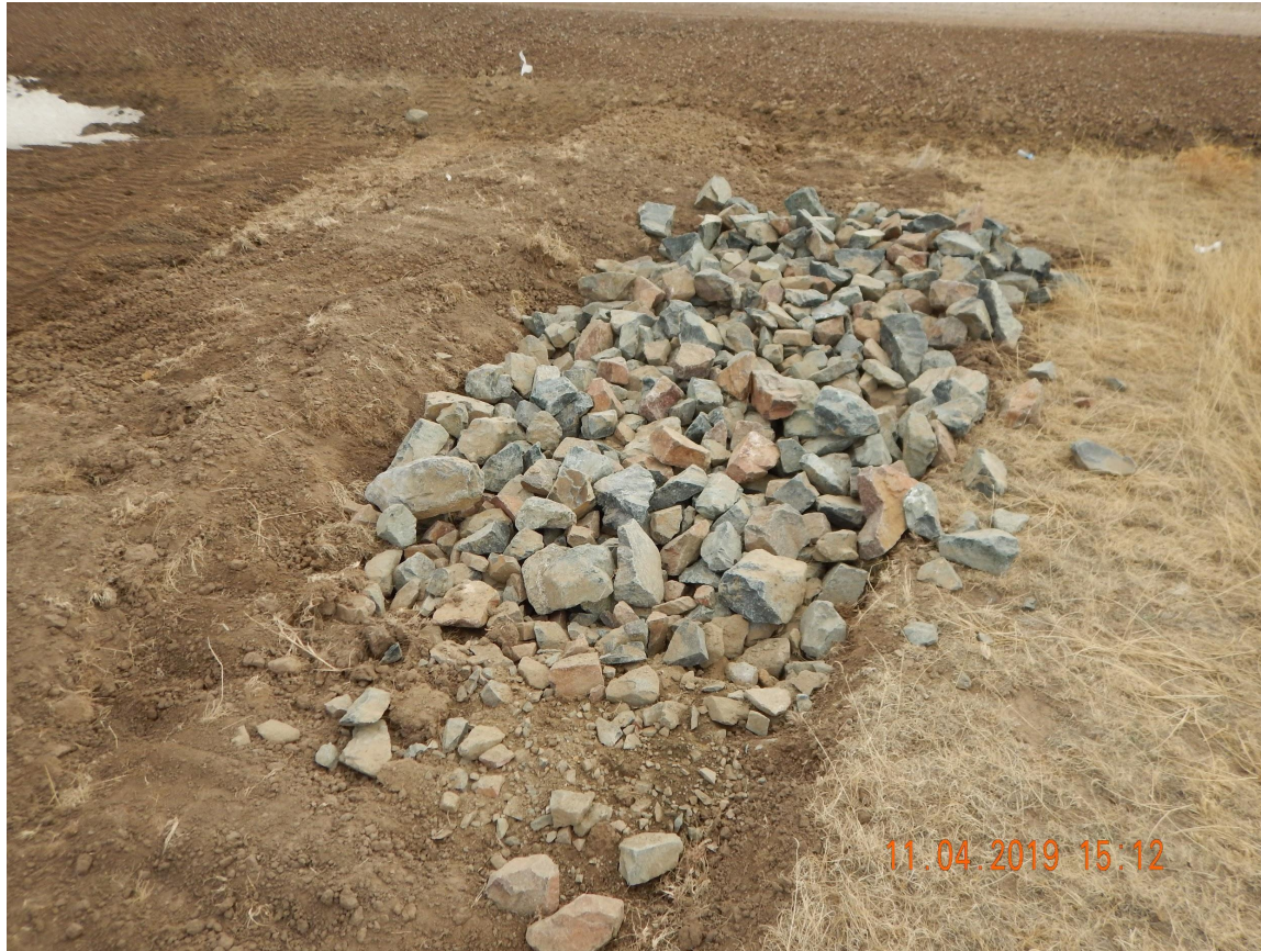
Photo 7. Photo taken from the southwestern perimeter of location (north of the access road), facing South. Photo illustrates an ~3'x6' area of riprap at the end point of the ditch. This would not be considered a sediment trap.
