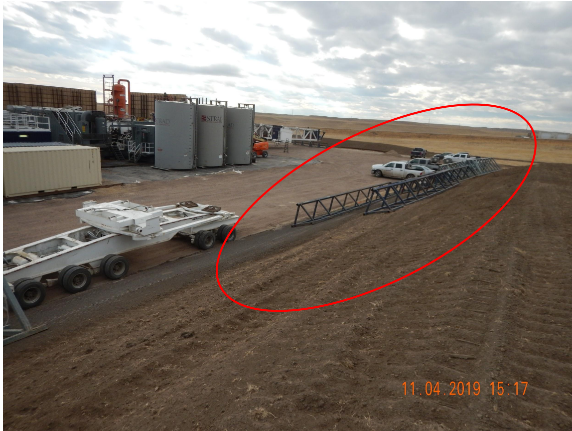
Photo 12. Photo taken from the northern topsoil stockpile, facing West. Photo illustrates equipment being stored on the topsoil stockpile which should be prohibited.
