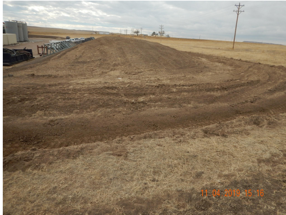
Photo 11. Photo taken from the northeastern perimeter of location, facing West. Photo illustrates the second topsoil stockpile which has been temporarily stabilized with equipment tracking.
