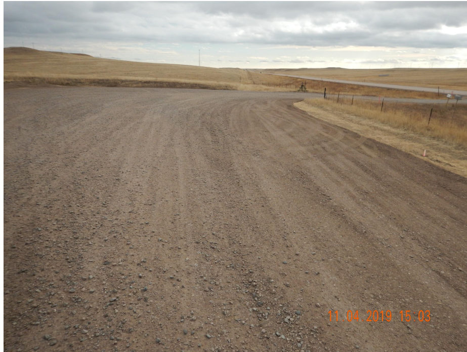
Photo 1. Photo taken from the entrance of location off HWY 85, facing South. Photo illustrates Operator has constructed and gravelled an access road.
