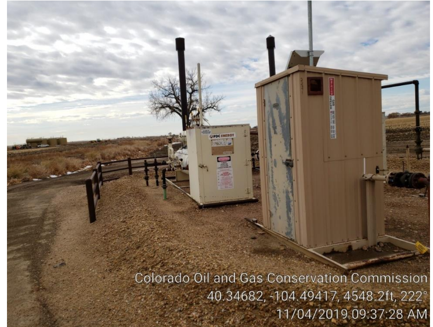
Photo #3 Separator & Meter Run
