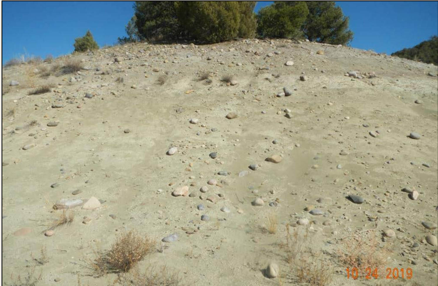
Photo 4. View of bare and eroding soils on the well pad cut slope.
