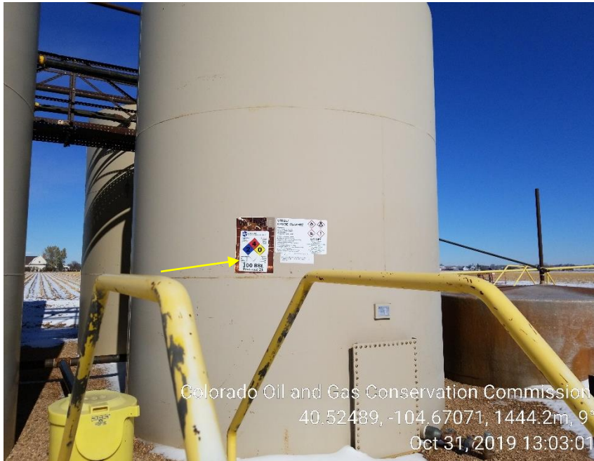
Photo 5: Labeling added to south tank
