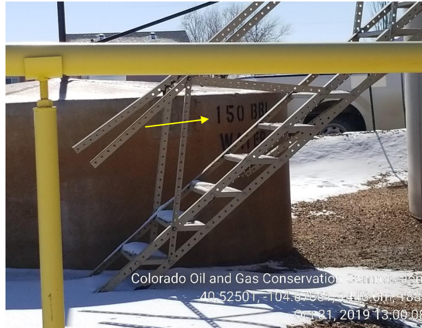
Photo 11: BBLS on wrong side of tank.
