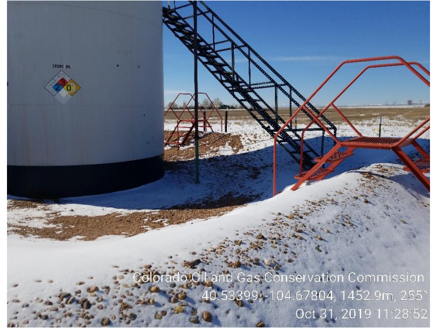
Photo 4: Weeds removed, hole repaired
