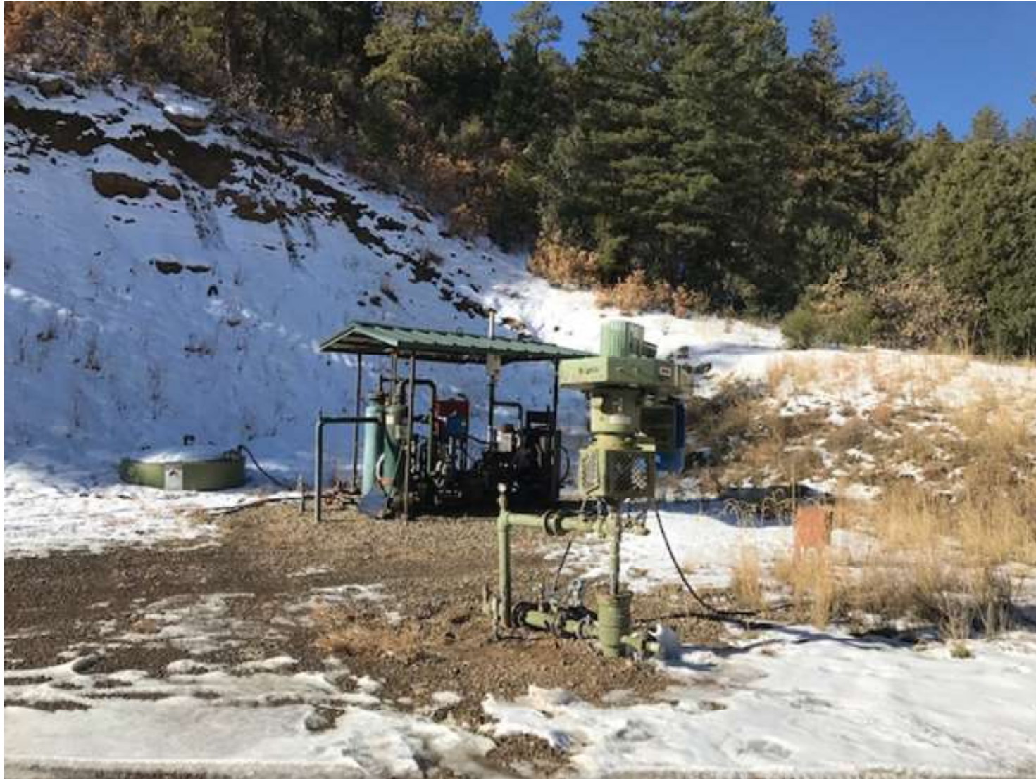
PHOTO 1: REPLACED THE PACKING TO STOP THE WATER LEAK. PACKINGS WERE SECURELY FASTENED.
