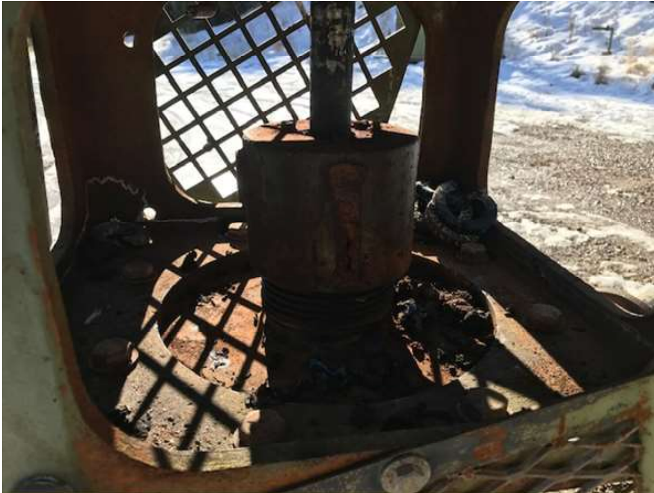
PHOTO 2: REPLACED THE PACKING TO STOP THE WATER LEAK. THE NUT OVER THE PACKING WAS SECURELY FASTENED.
