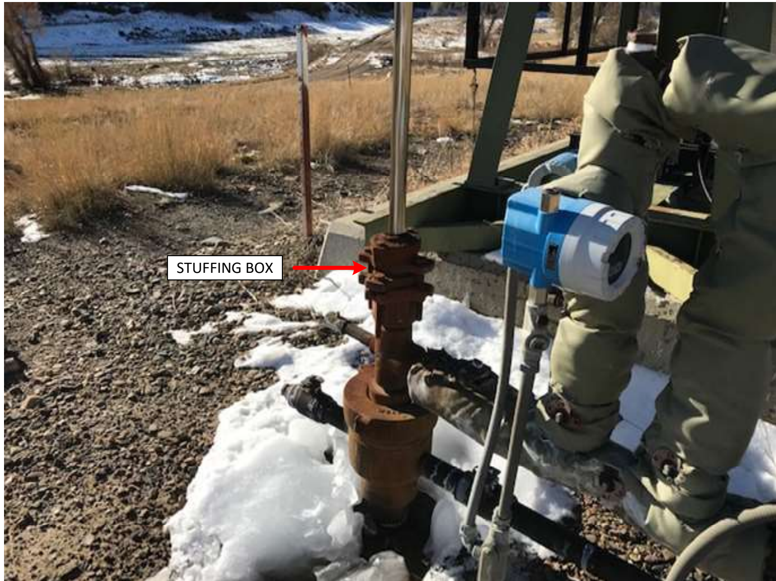
PHOTO 1: REPLACED THE PACKING TO STOP THE WATER LEAK. THE STUFFING BOX WAS SECURELY FASTENED.
