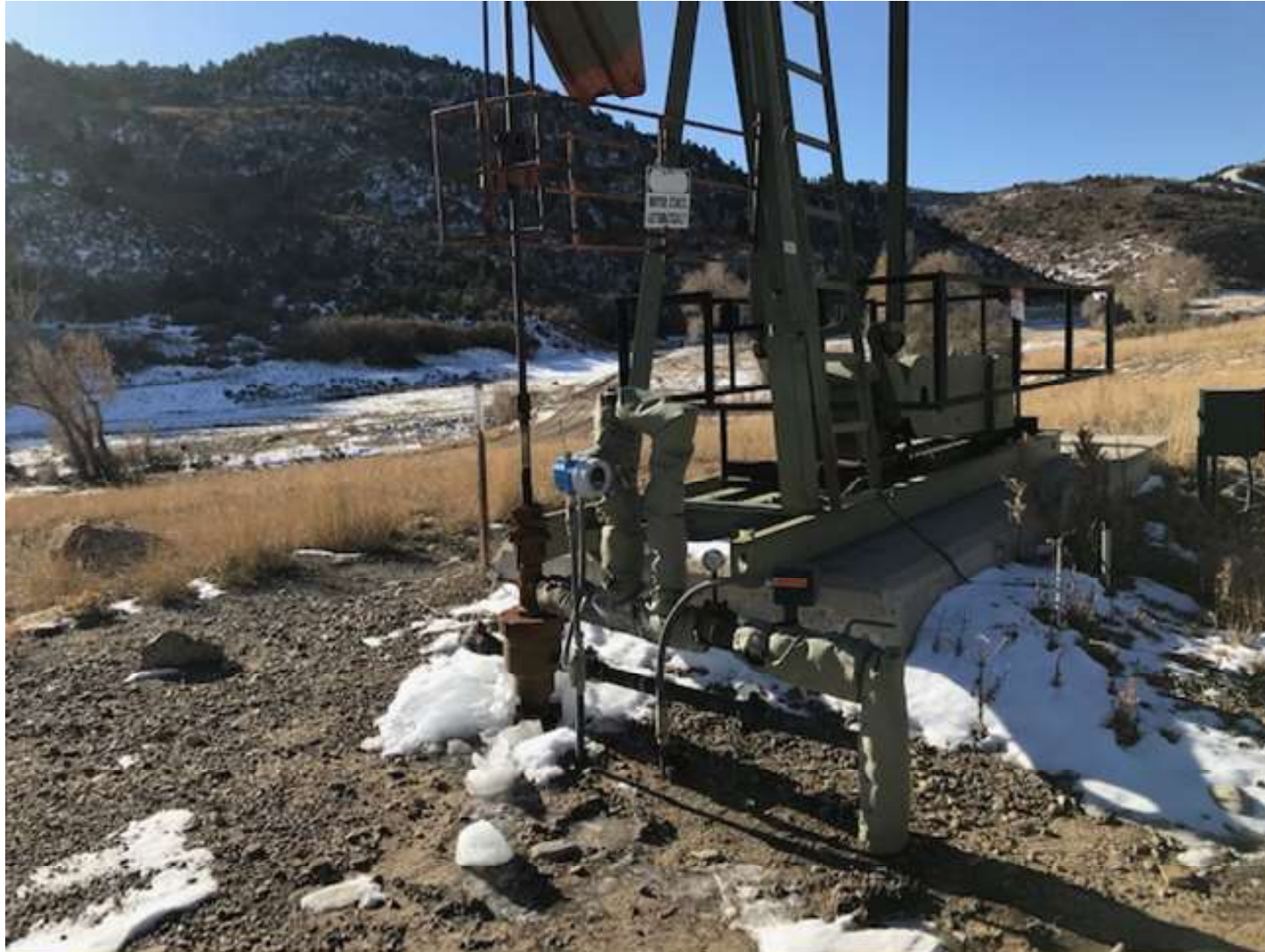
PHOTO 2: REPLACED THE PACKING TO STOP THE WATER LEAK. THE STUFFING BOX WAS SECURELY FASTENED.
