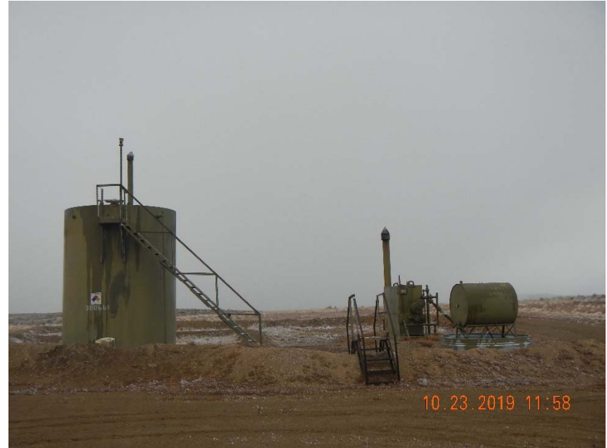
Photo 2. Approximately 18 foot setback between separator and heated crude oil tank.
