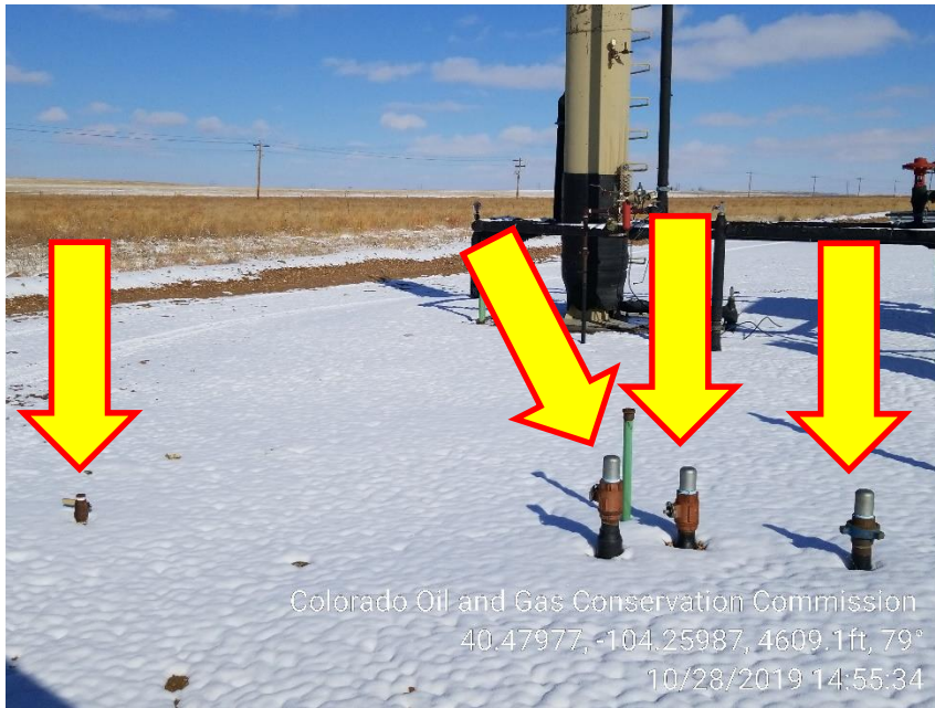
Photo 3 – Unmarked 1" and 2" Risers
