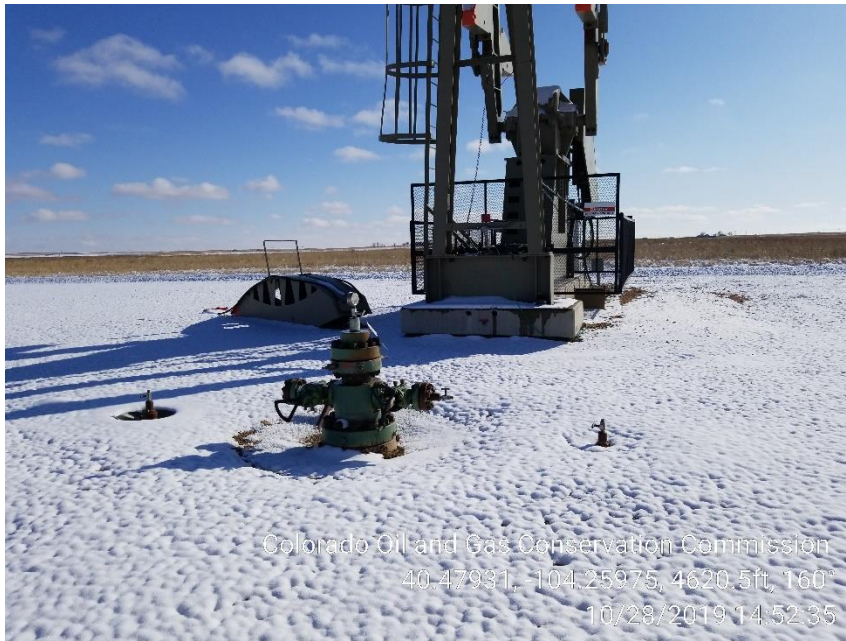
Photo 1 – Wellhead TA'd
