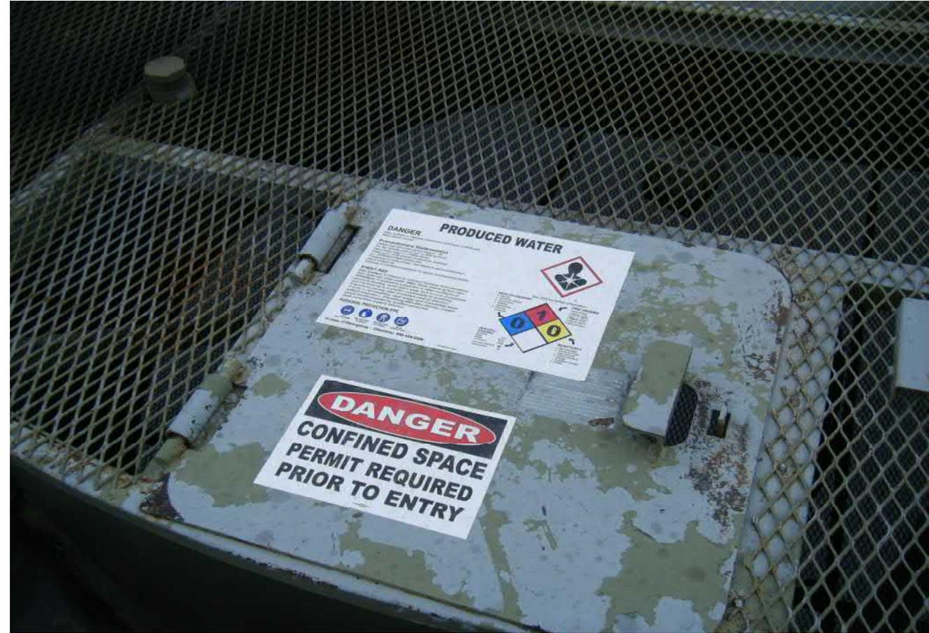
The 80 bbl. fiberglass open top tank has been labeled to comply with Rule 210.d.
