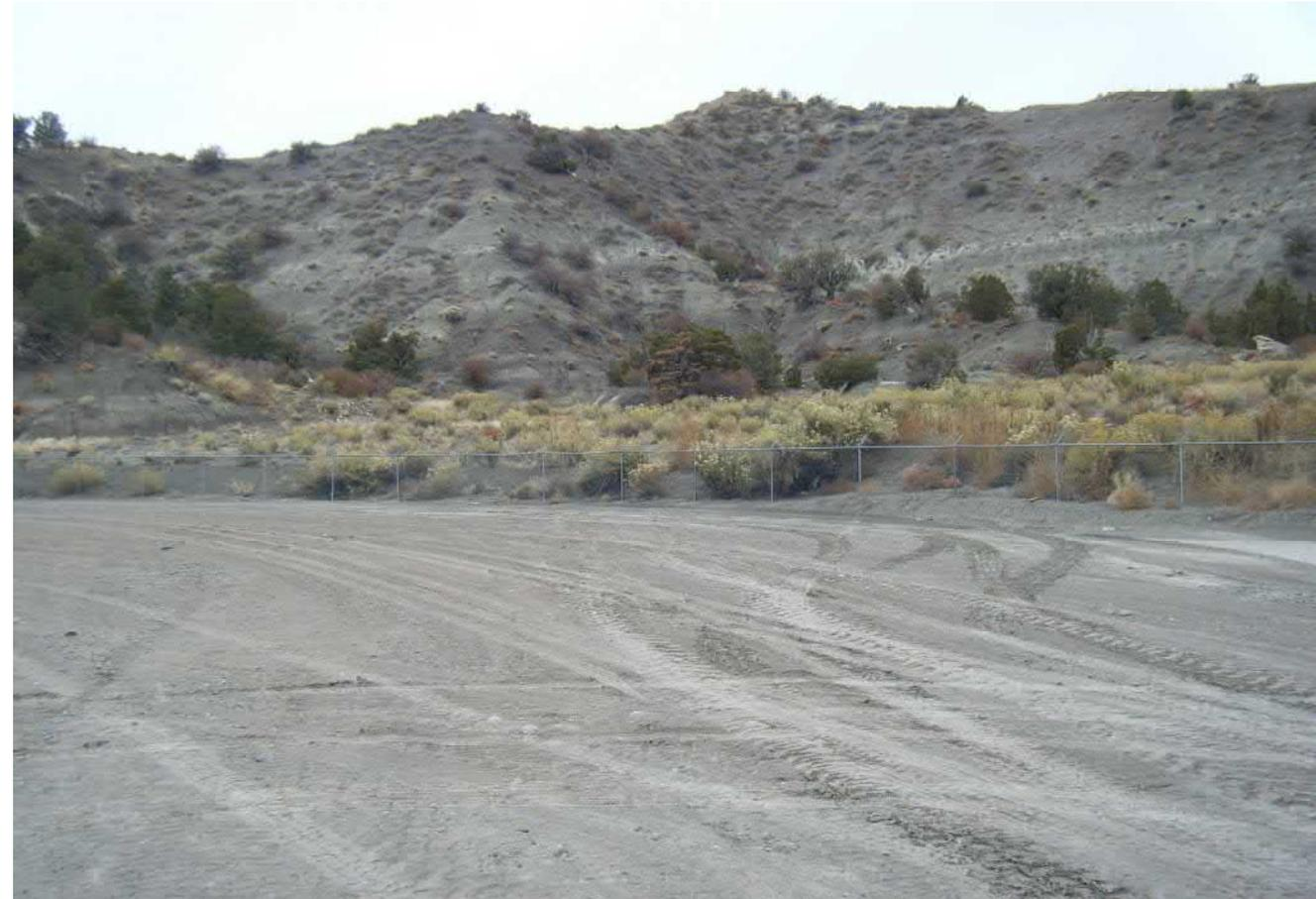
Storm Water management controls have been maintained and established to stabilize storm water run on and run off. Cleaned the diversion around the upper level facility and established a drainage diversion along southern edge of the upper level facility to stabilize erosion and site degradation to comply with Rule 1002.f.
