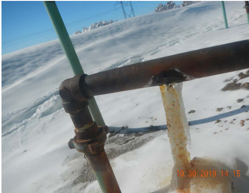
Photo #3 ongoing spill at tank battery
