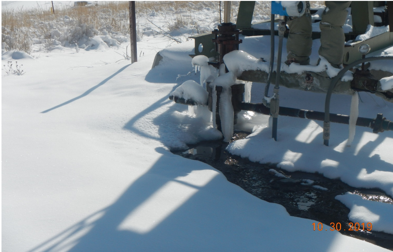
Photo 1. There is water leaking from the well head. There is ice buildup around the wellhead and water dripping.
