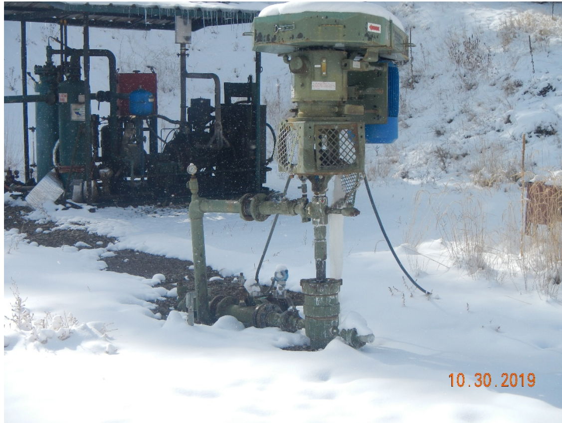
Photo 1. There is water leaking from the well head. There is ice buildup around the wellhead and water dripping. Corrective action was not properly performed.
