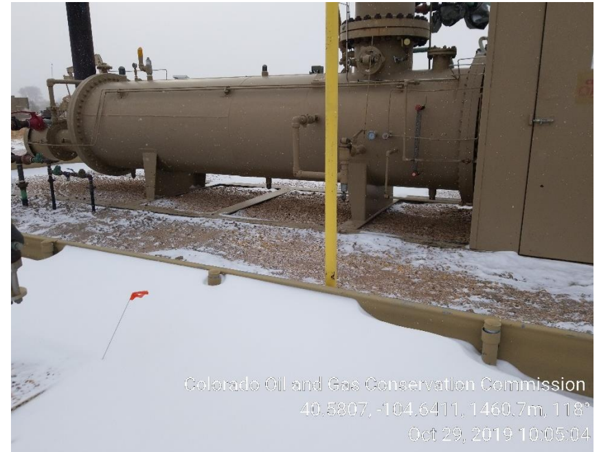
Photo 4: Separator not anchored
