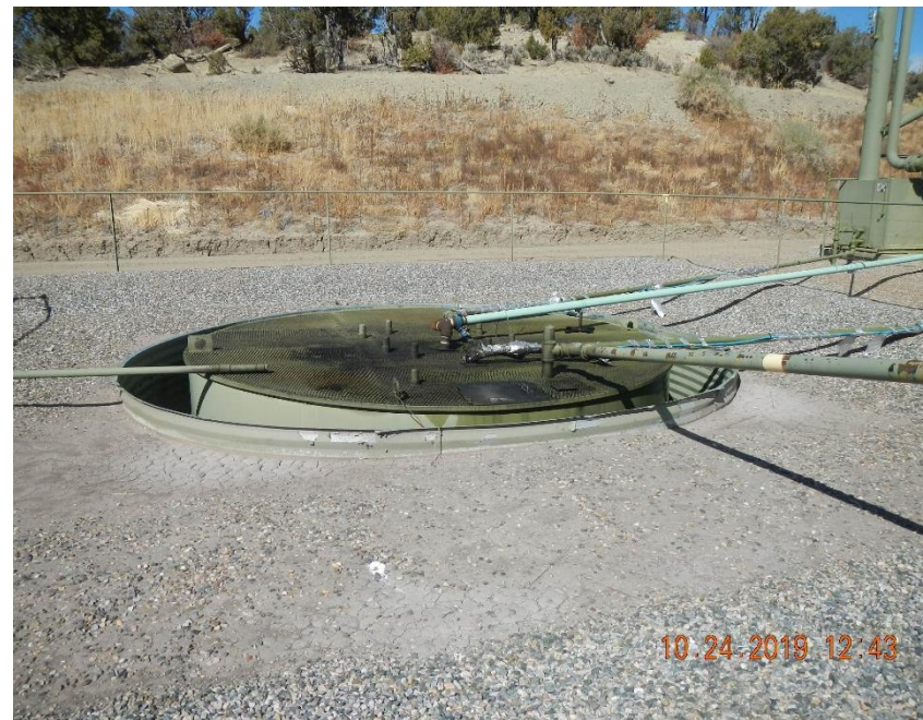
Open topped below grade tank is not labeled.
