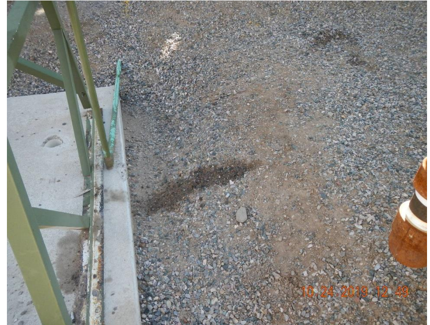
Stained gravel beneath valve on lube oil container.
