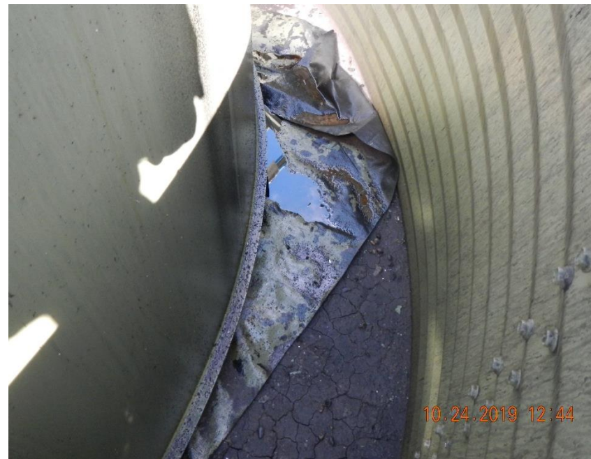
Fluids and stained soil present within cellar for below grade tank.
