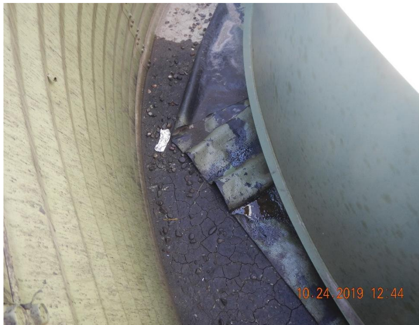
Soil within cellar for below grade tank is wet and stained.
