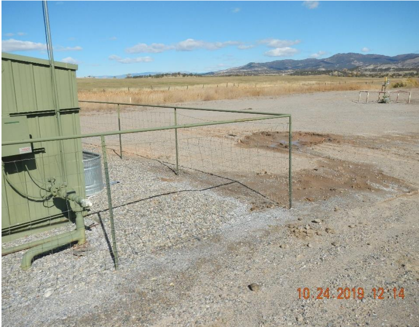
Damp area on location from separator to low spot on location.
