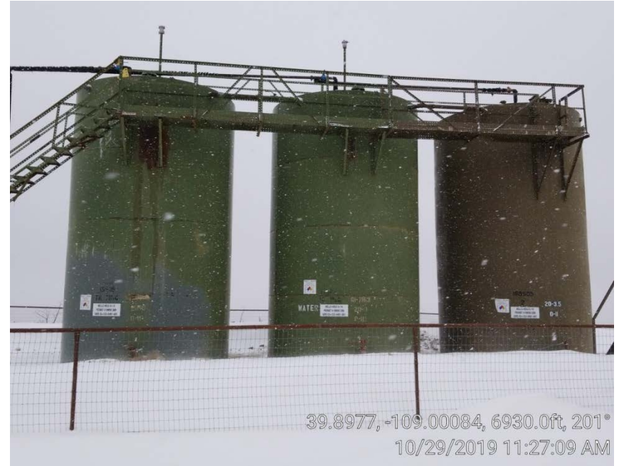
Photo 3. Tank battery.
