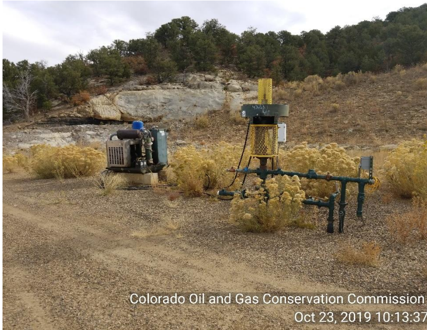
Photo 3 Motor skid is reconnected to PC pump on well head. Weeds on location and around equipment
