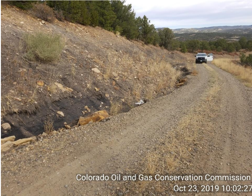
Photo 3 BMP's not in place to control erosion on access road to location. Ditch is approx. 3ft wide in places.
