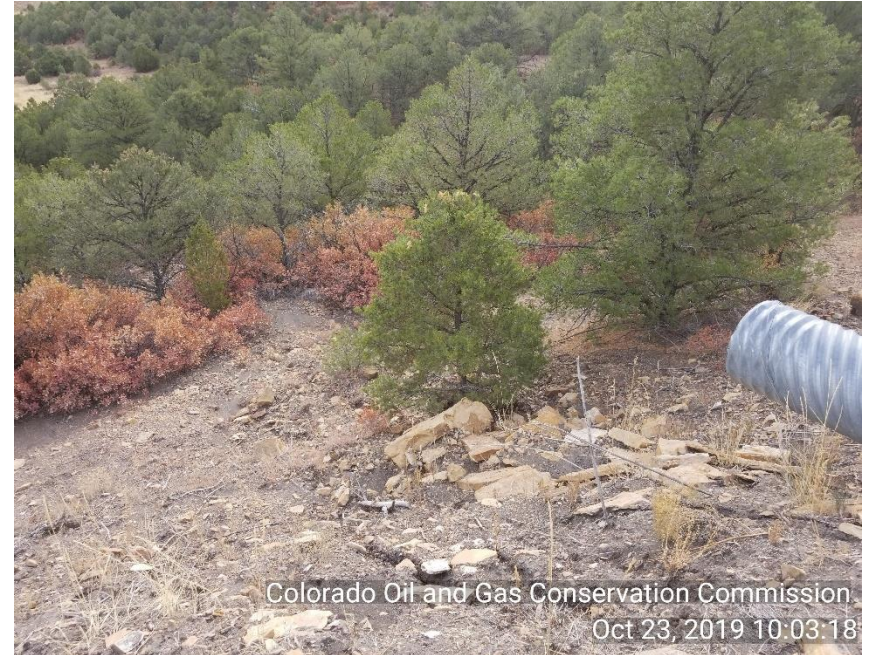
Photo 4 Sediment from Pic 3 erosion BMP issues not controlled and being carried off rightaway.
