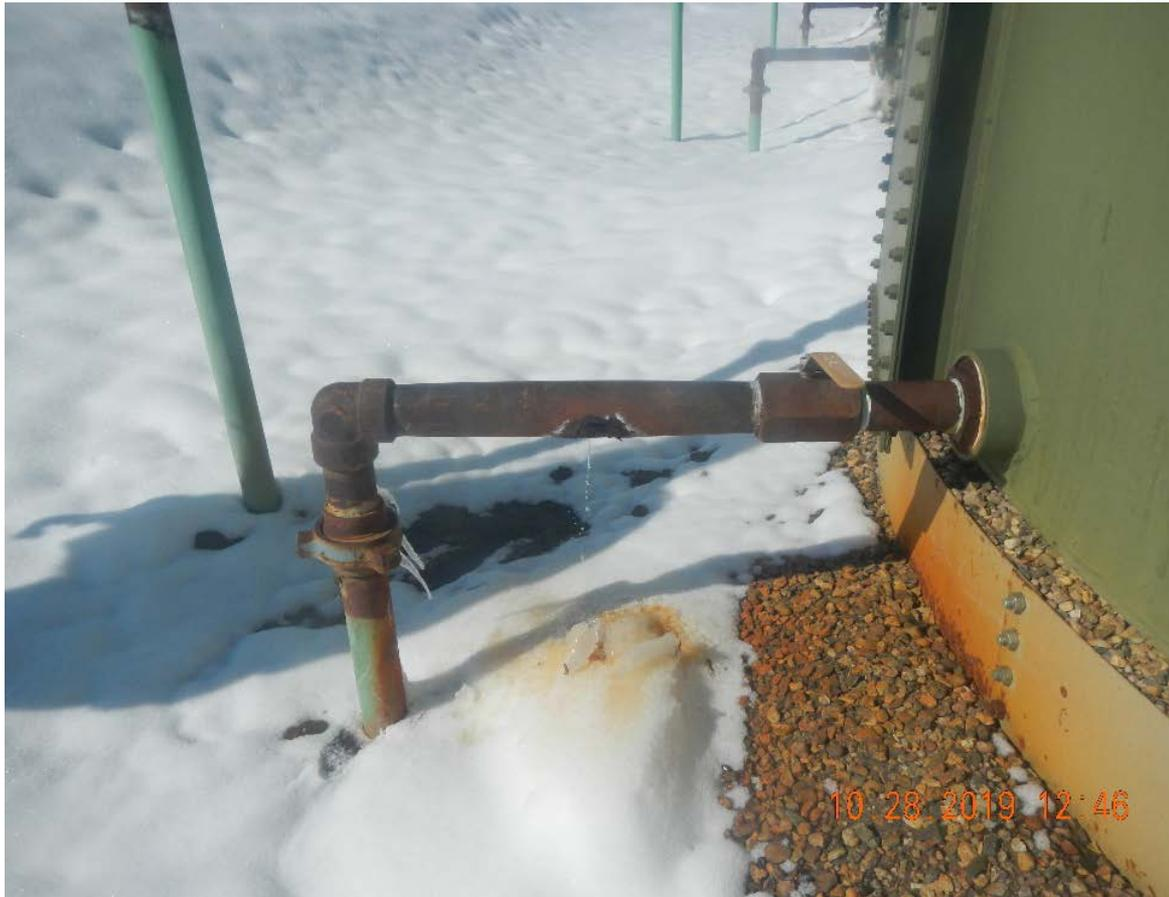
Photo #8 ongoing spill at tank battery
