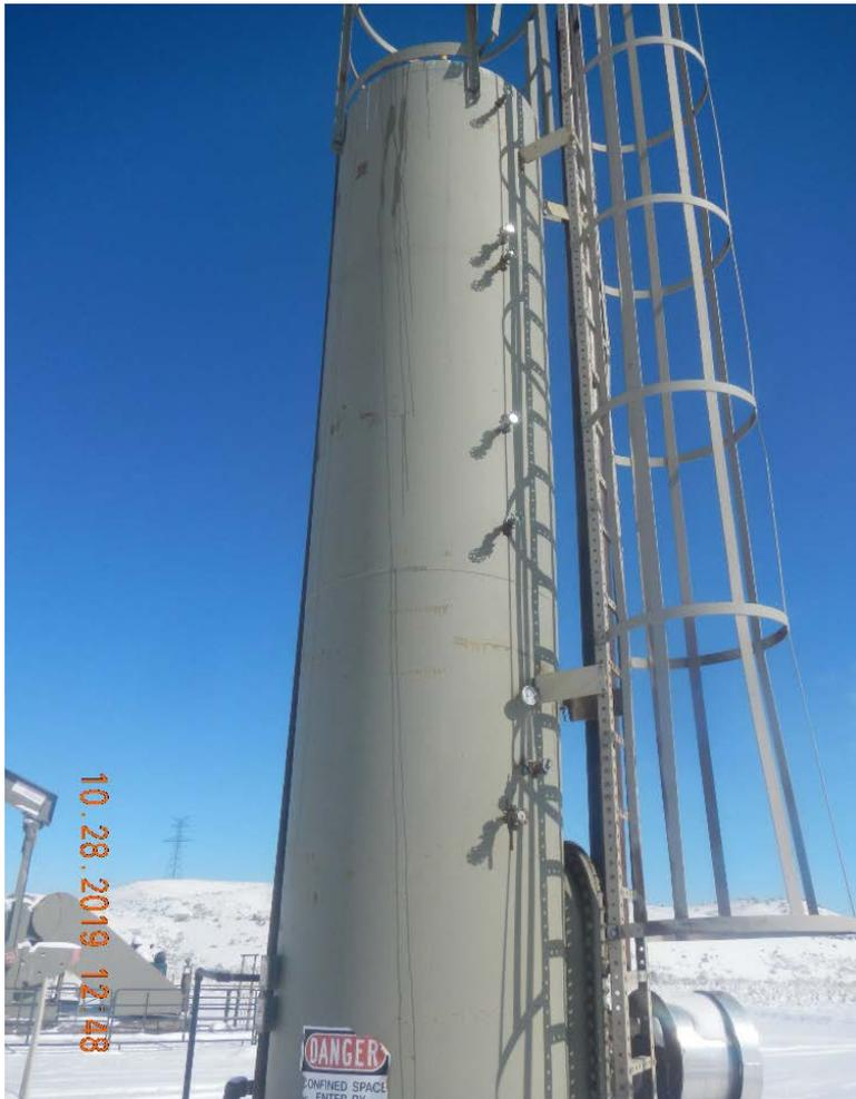
Photo #14 Treater. The sight glass that had caused a spill previously has not been replaced.
