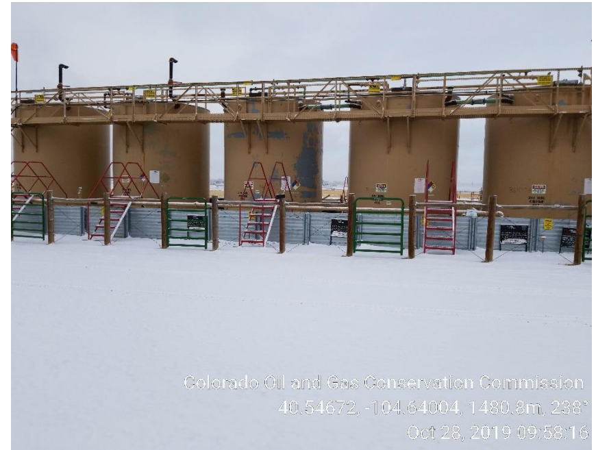
Photo 2: Tank Battery
