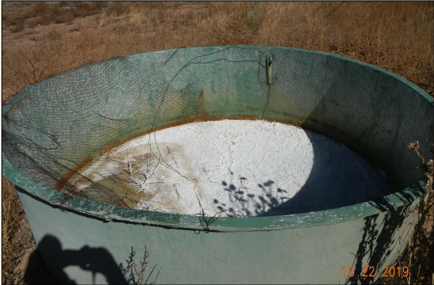
Photo 2. View of tank that remains on the location. Unknown white material remains on the bottom of the tank.
