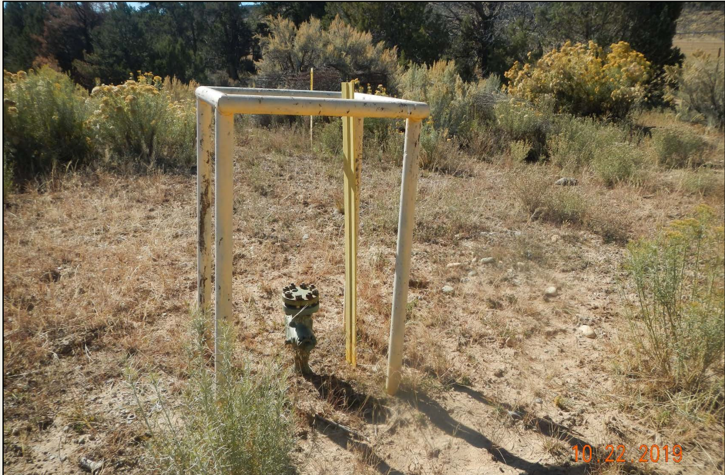
Photo 3. View of riser that remains on the location.
