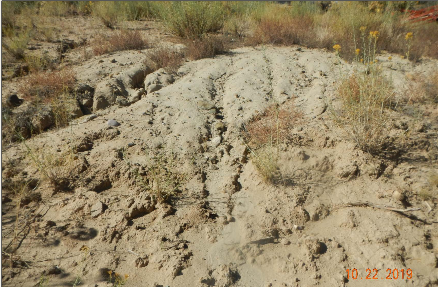
Photo 7. View of erosional channels in the northeastern fill slope, upstream from sediment deposition shown in Photo 6.
