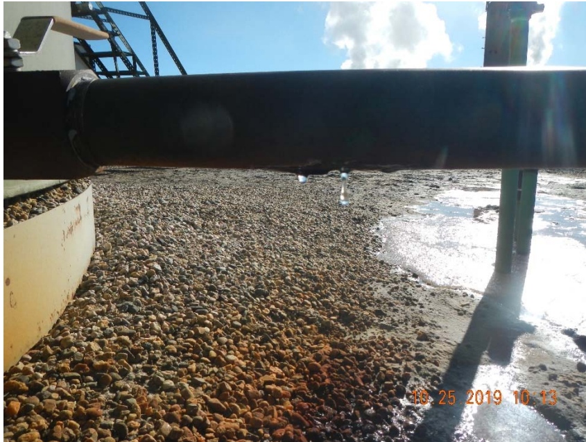
Photo 3. Ongoing leak at tank flowline, water in photo is all from leak.
