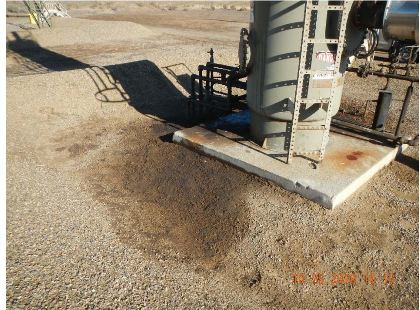
Photo 6. Stained soil at separator.
