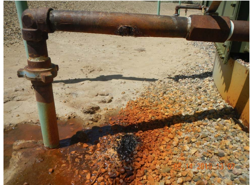
Photo 4. Ongoing leak at tank flowline. Photo from 8/14/2019 inspection document number 689802979.
