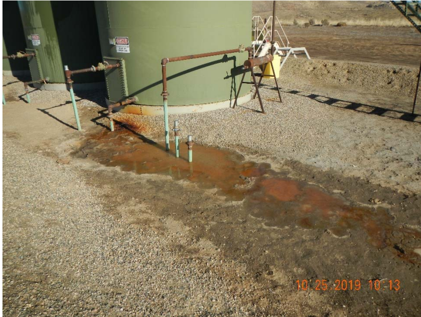
Photo 5. Ongoing leak at tank flowline, water in photo is all from leak.
