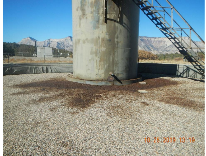
Stained gravel inside of tank containment berm.
