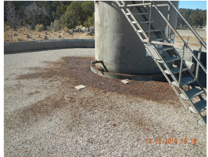
Stained gravel inside of tank containment berm.
