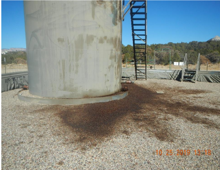
Stained gravel inside of tank containment berm.
