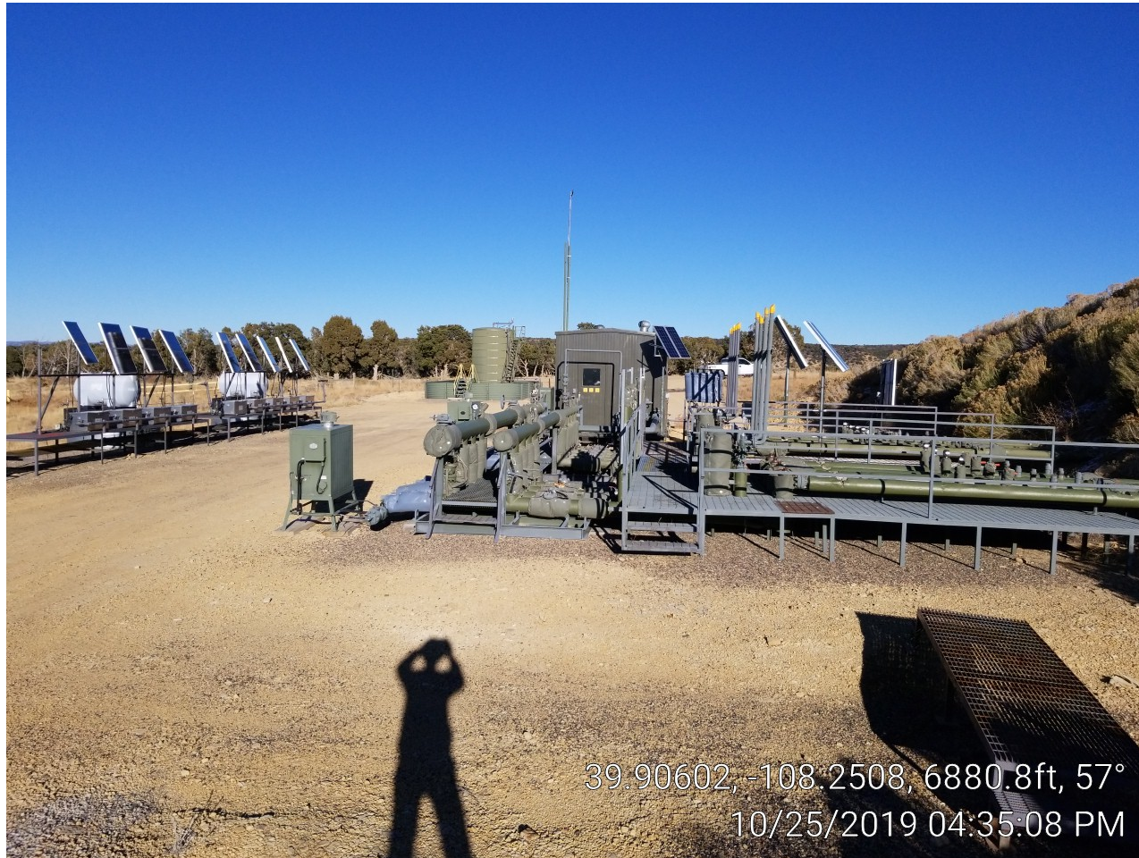
Photo 2. Header, chemical, separator, and tank battery.
