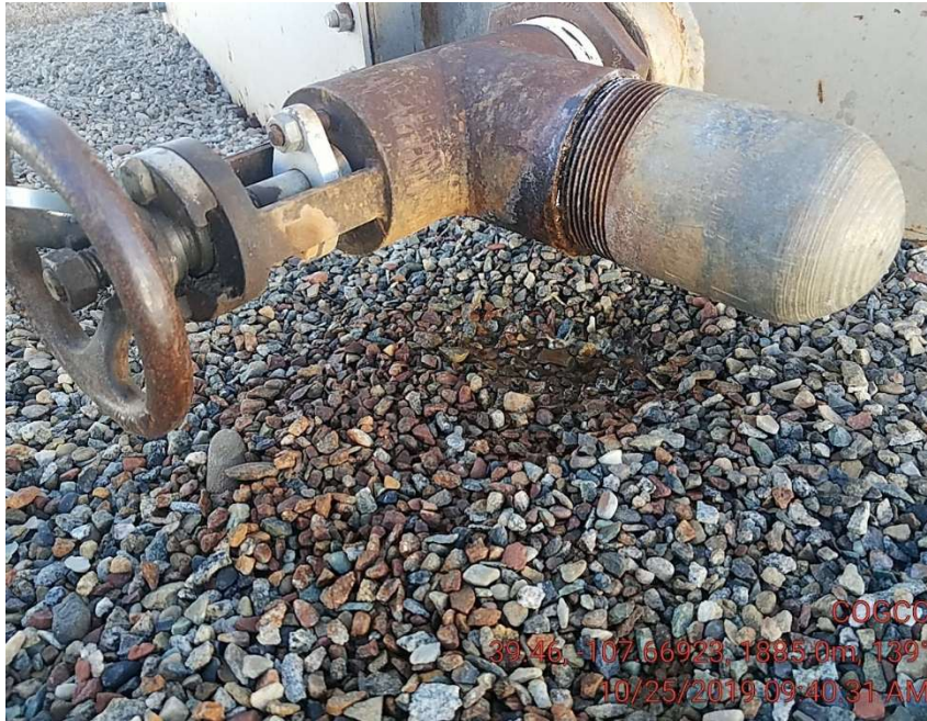
Leaking load out valve
