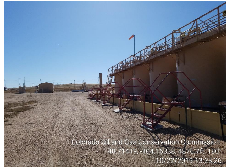
Photo 2 – Tank Battery
