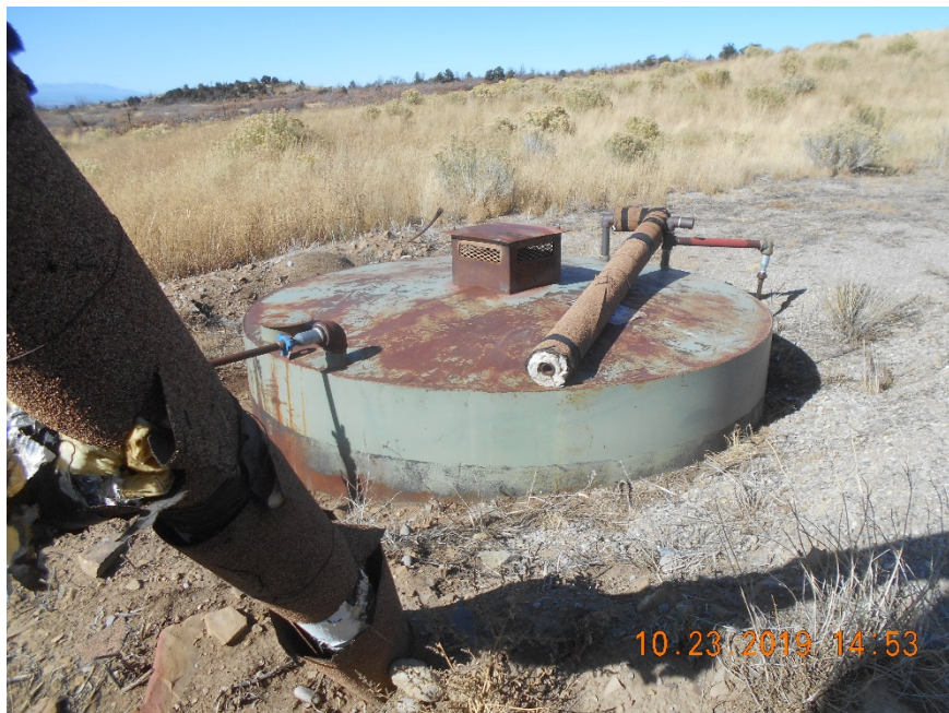
Reboiler tank with disconnected line
