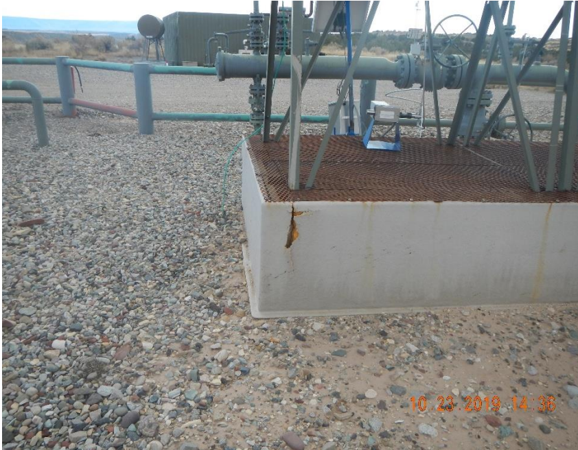
Damaged fiberglass secondary containment
