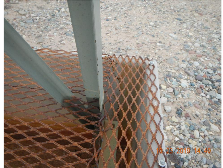
Damaged fiberglass secondary containment
