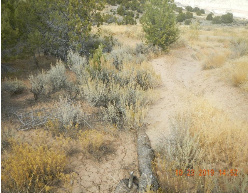
Unmaintained waddles along ditch.
