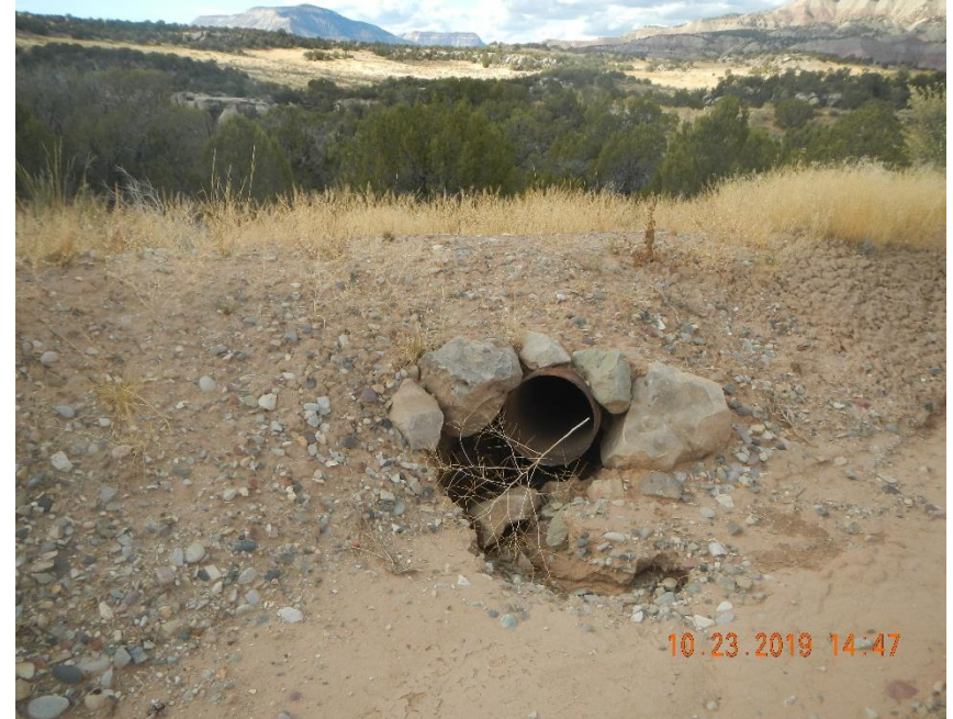
Washed out around drainage pipe.
