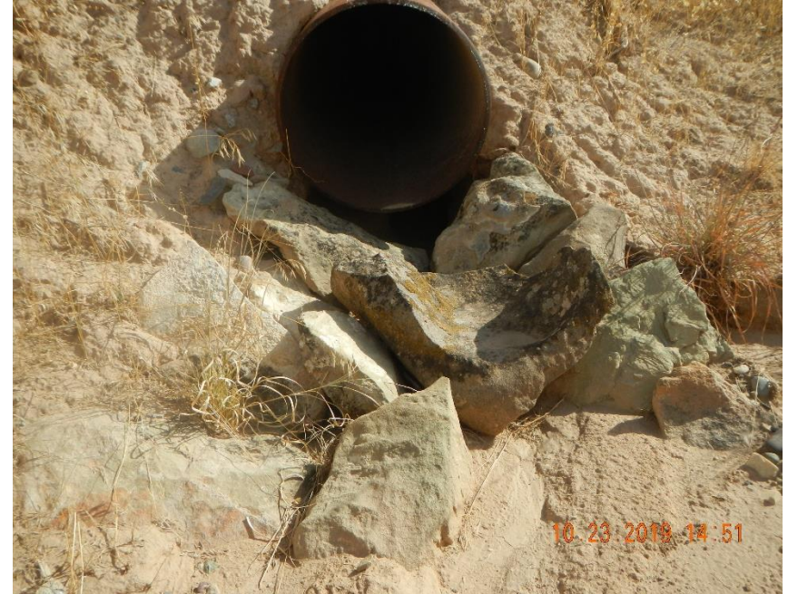
Washed out around drainage pipe.
