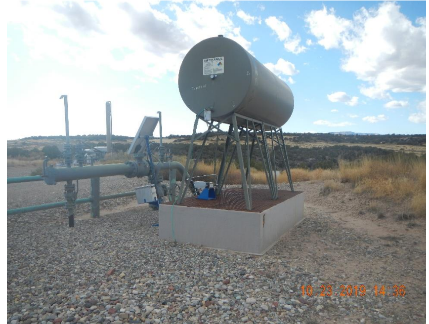
Damaged fiberglass secondary containment
