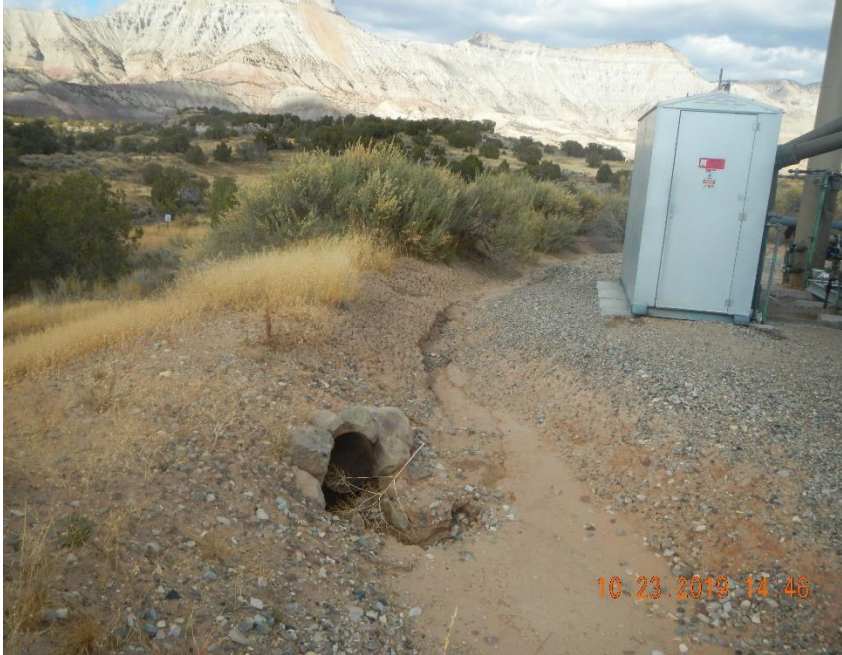
Washed out around drainage pipe.
