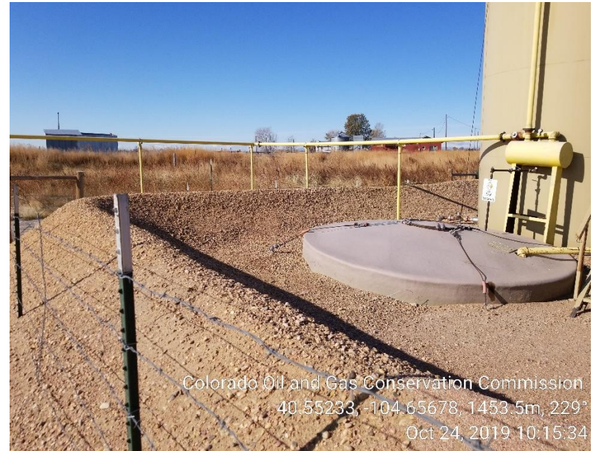
Photo 4: Holes in berm repaired.
