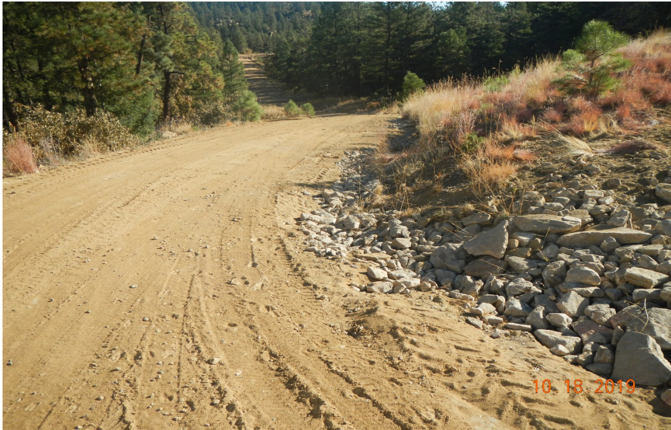
Photo 3. Rock rip/rap was installed along the rad near the location.
