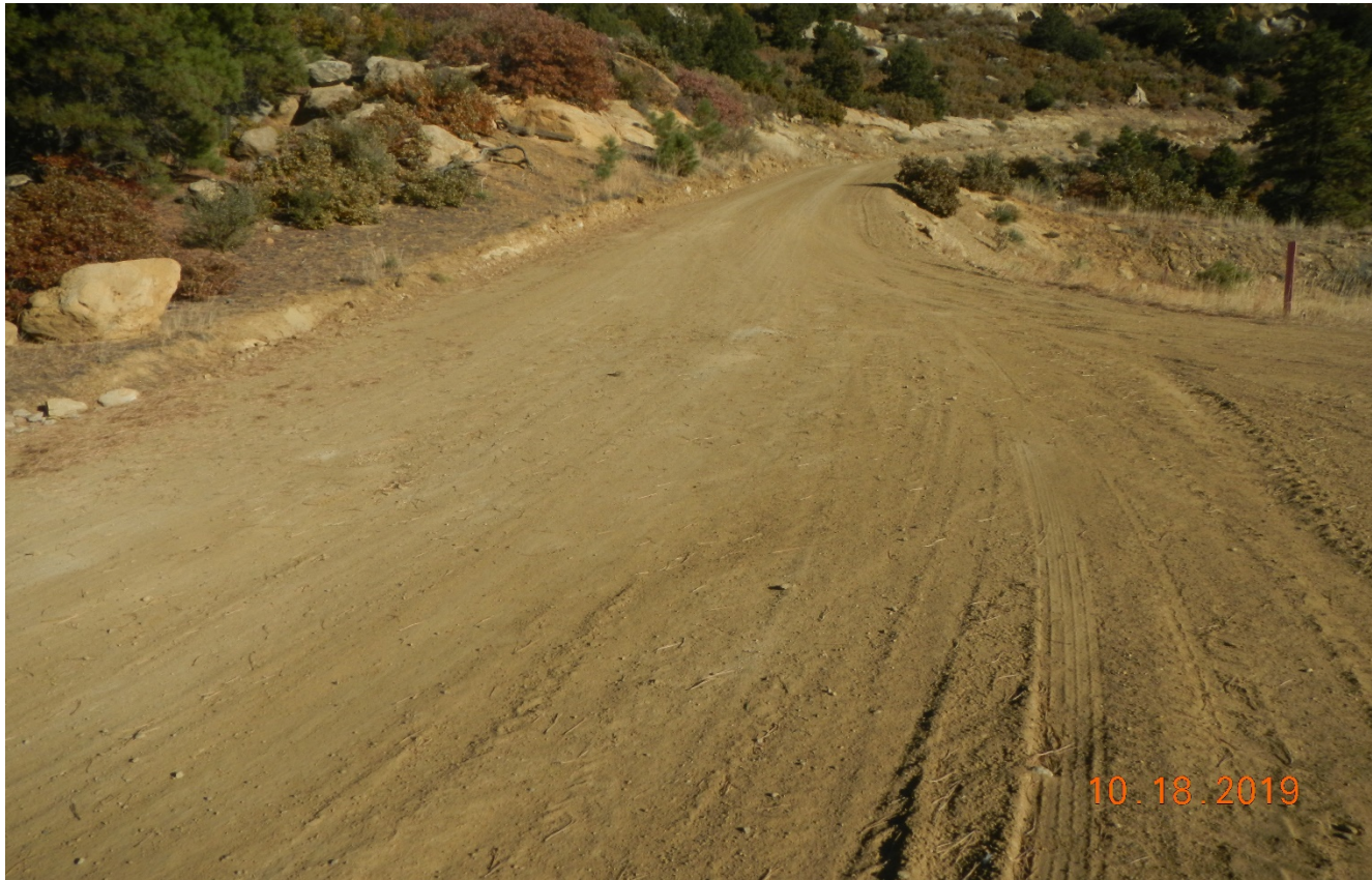
Photo 1. The main road has been regraded.
