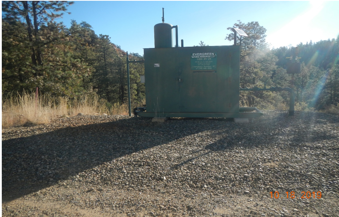
Photo 3. Facing at the location. Sign is installed.
