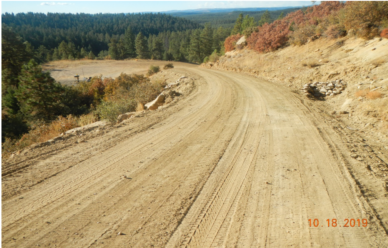
Photo 1. The main road has been regraded. The culvert has been maintained.
