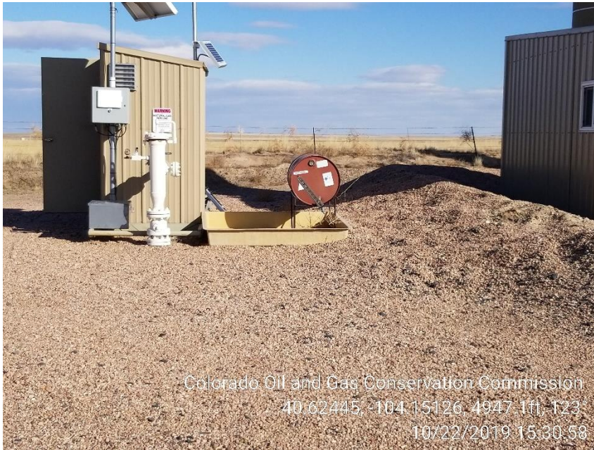
Photo 3 – Unused Methanol Tank and Containment
